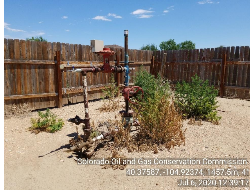
Photo 4: Wellhead; WEEDS
