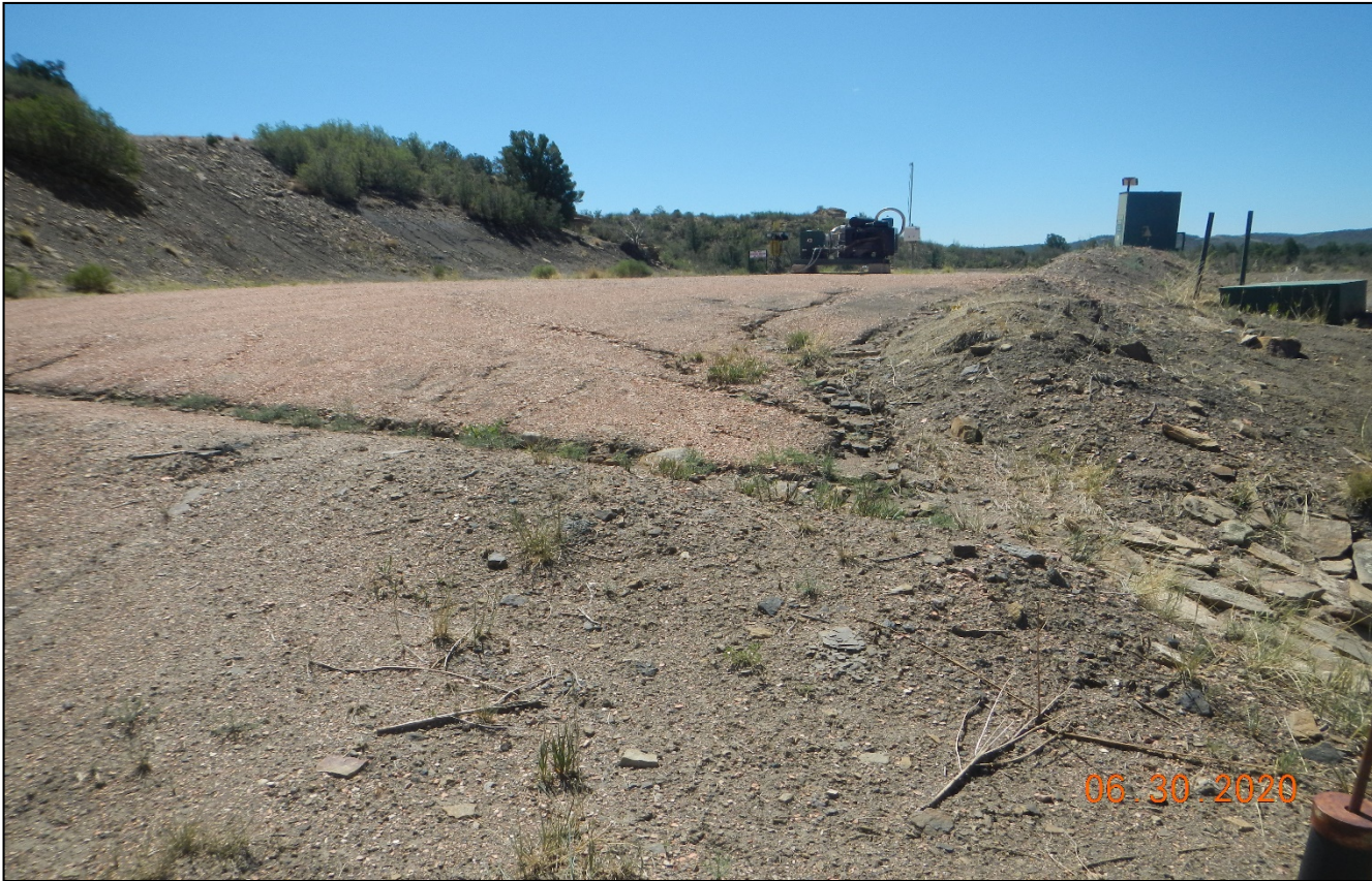
Photo 5. Facing toward the location. There is signs of stormwater erosion off the pad which is directed to a sediment trap shown in the next photo.
