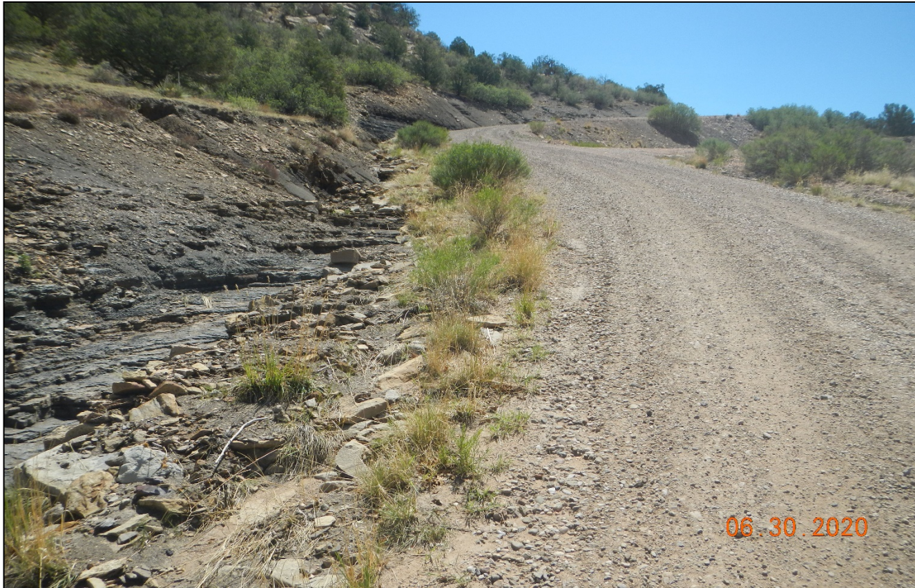
Photo 4. Facing east along the access road. There is a long stretch of road which does not have culverts or BMP's which is contributing to the volume of stormwater directed to the culvert shown in previous photo.
