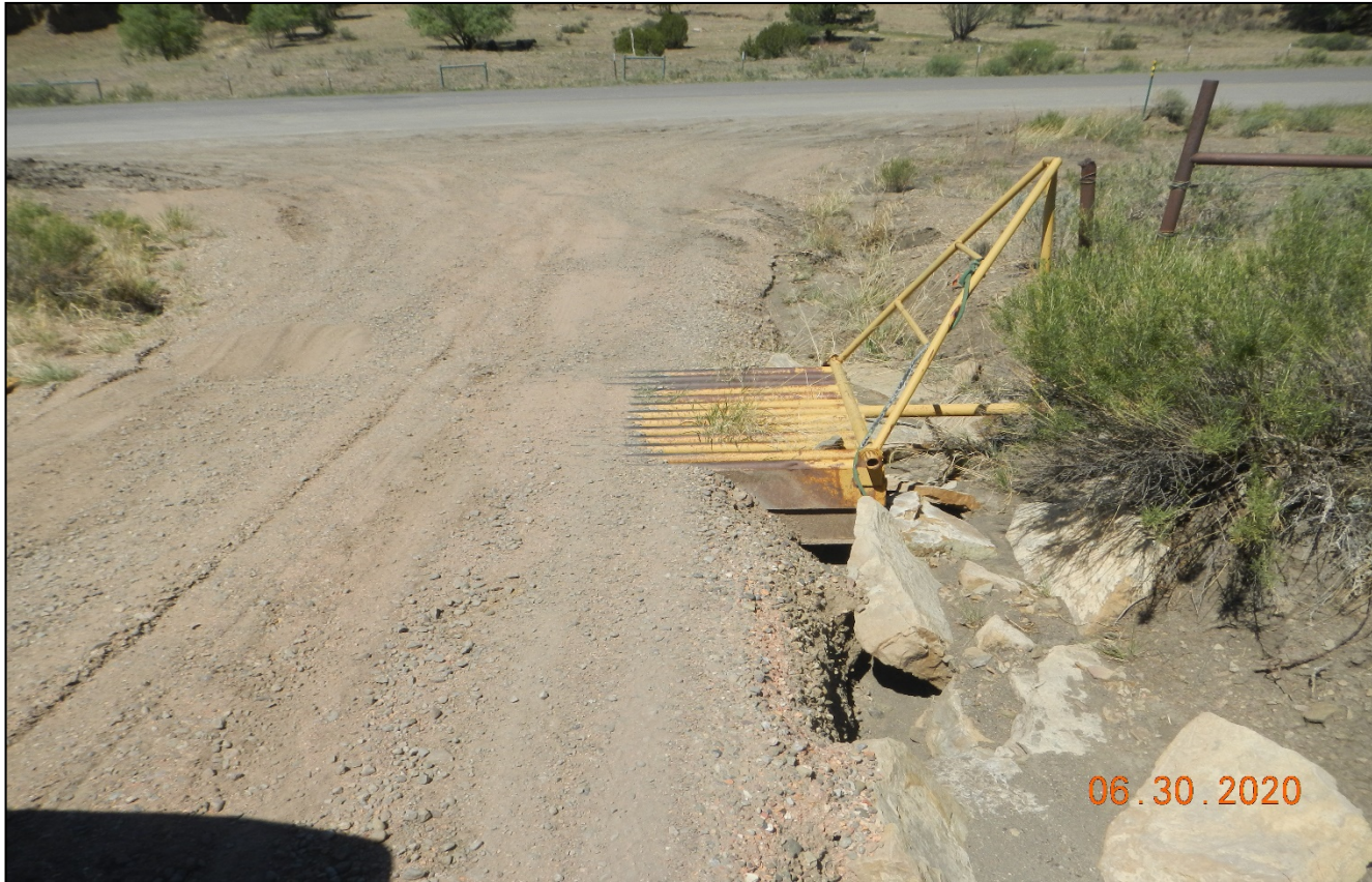
Photo 2. There is erosion occurring along the side of the cattleguard and the cattleguard is filled in with sediment.
