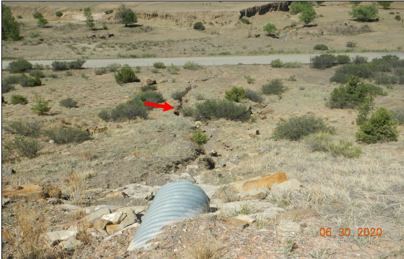
Photo 3. Facing southwest toward the culvert outlet. Stormwater is causing erosion which is directed toward the county road.
