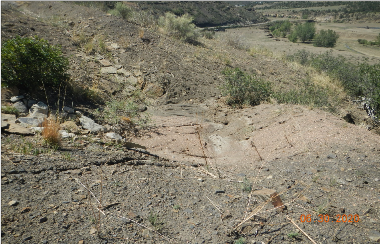
Photo 6. The sediment trap is full of sediment.
