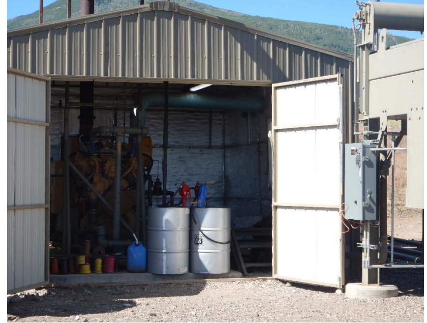
Photo #14 – Open shed in southeast end of pad. Note 55-gallon drums slightly overhang cement foundation of shed. Operator was notified via phone of this issue on 7/3/2020.
