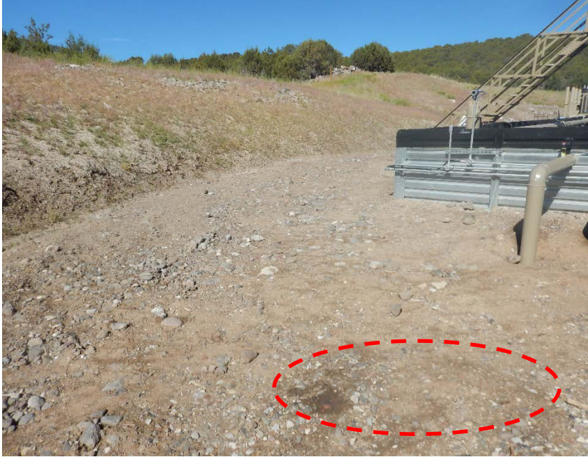
Photo #13 – Localized accumulation of oil-stained soil southwest of tank battery.
