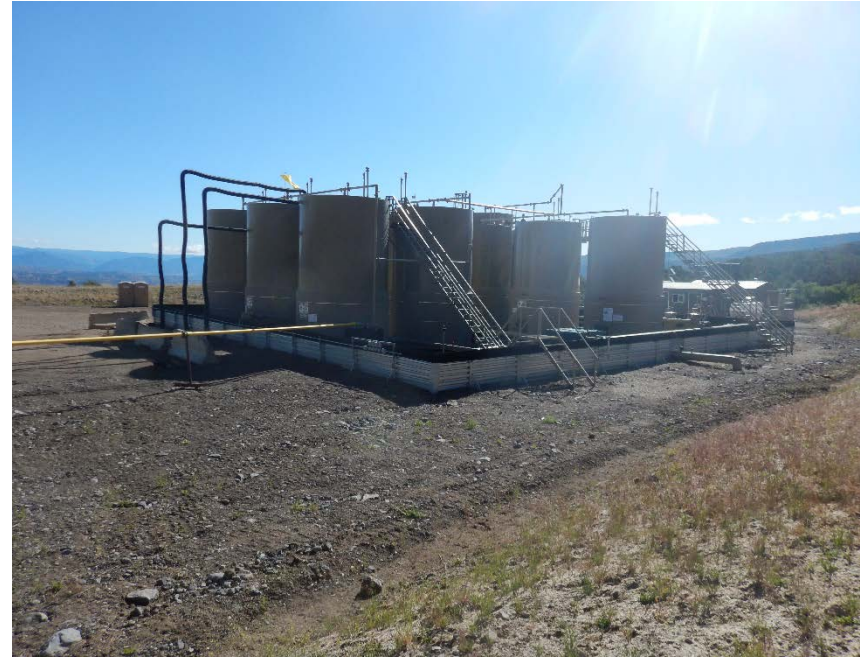
Photo #10 – Overview of tank battery from southwest. Photo depicts backfilled former excavation area for Remediation Projects #11661 and/or #11786.
