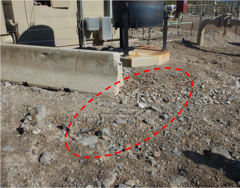
Photo #9 – Unused equipment (1/4" process pipe) located southeast of ECD. Photo depicts backfilled former excavation area for Remediation Projects #11661 and/or #11786.
