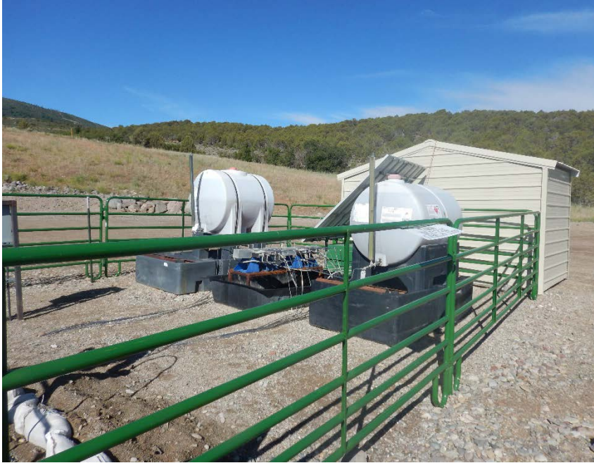
Photo #5 – View of day tanks and chemical pumps on west side of fenced wellhead area.
