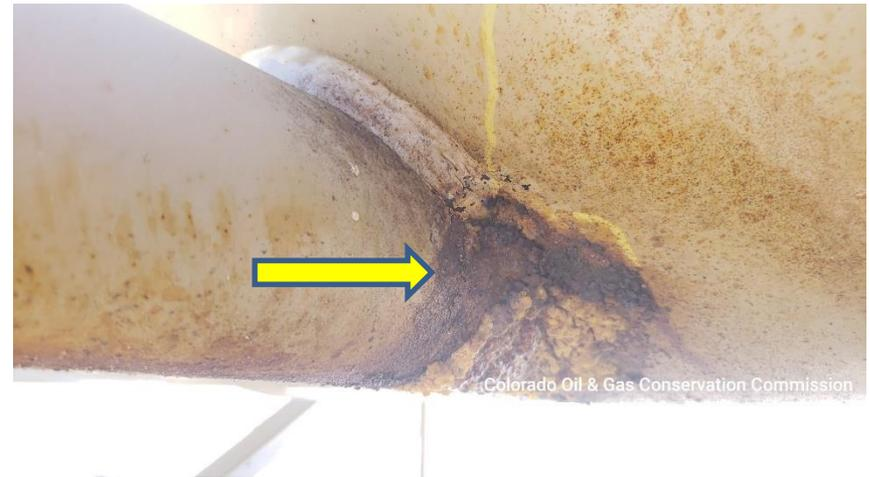
**Photo 5 Stained soil under east Horizontal Heated Separator**
