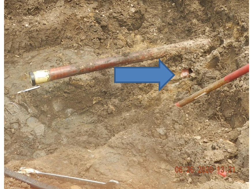
Close up view of South wall of excavation at Spill ID # 476987 with flowlines exposed; cut end of a second 3" fiberglass flowline can be seen between pipe stub and shovel handle. Date 6/26/2020.
