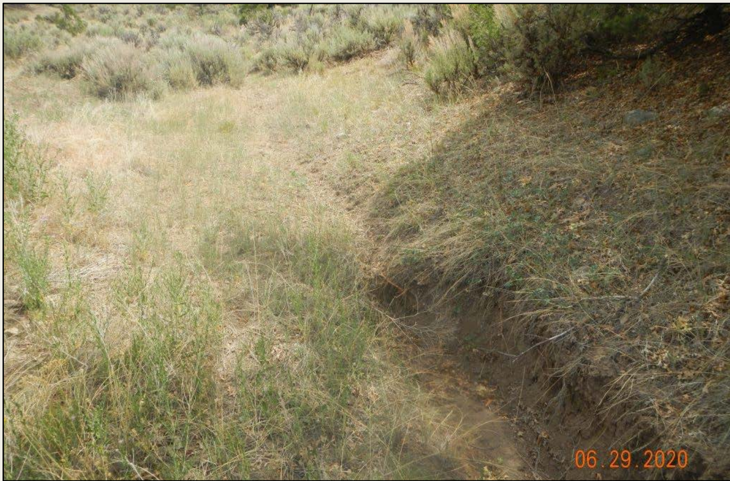
Photo 5. View of erosional headcut, approximately 3 feet wide and 2 feet deep, within the eastern stormwater diversion.
