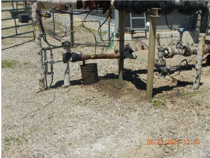
Photo 3. Stained soil at wellhead.
