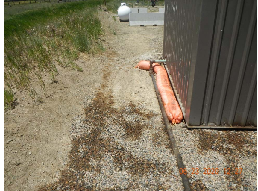
Photo 8. Stained soil from apparent spill.
