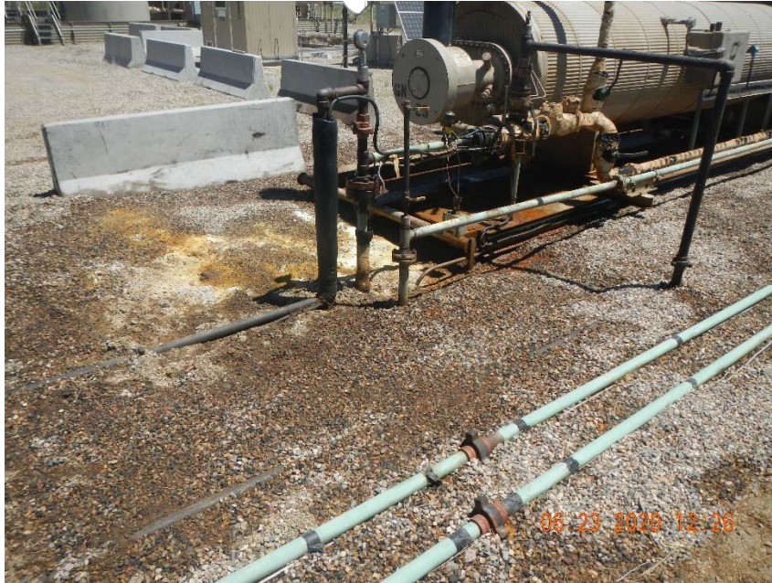
Photo 7. Stained soil from apparent spill.
