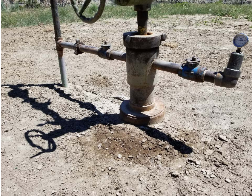
Photo #3 – Localized accumulation of oil-stained soil at wellhead.
