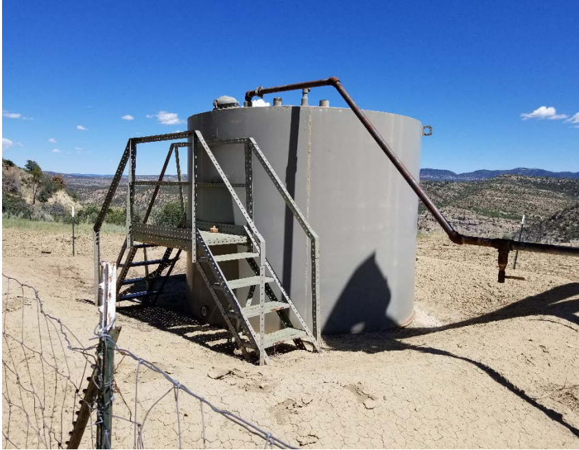
Photo #3 – View of tank from southeast. Note: berm is eroded.
