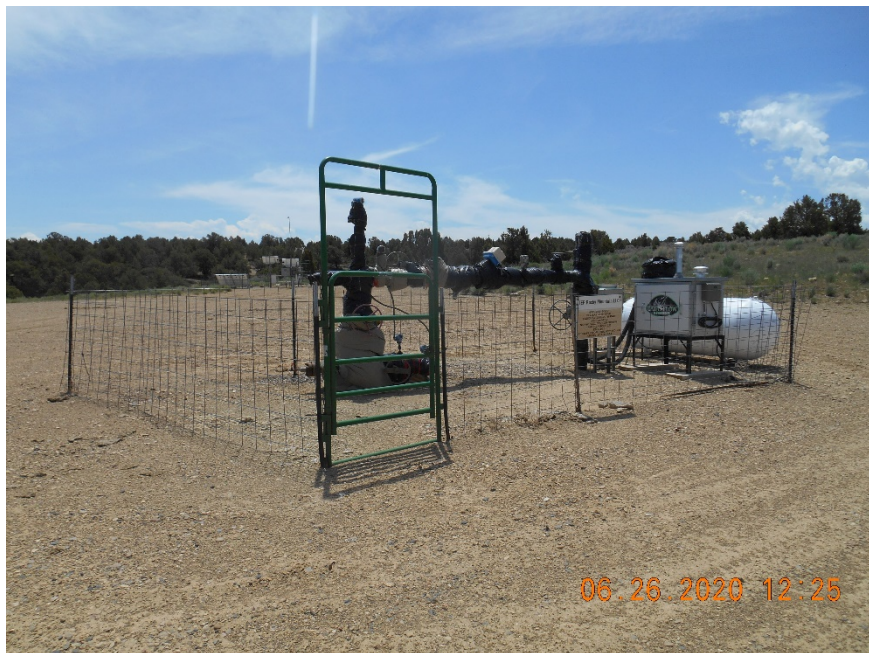
Injection wellhead & line heater
