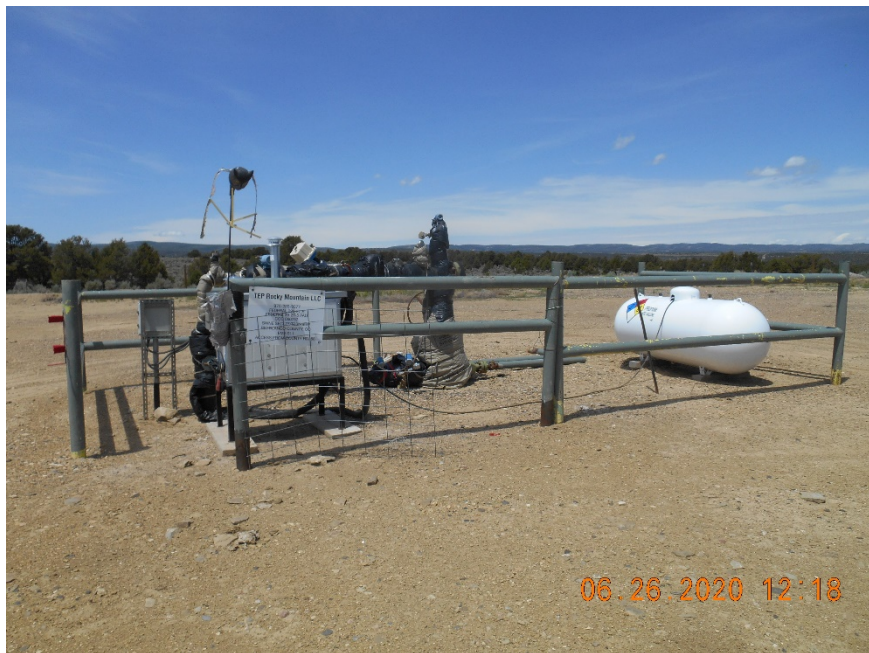
Injection wellhead & line heater
