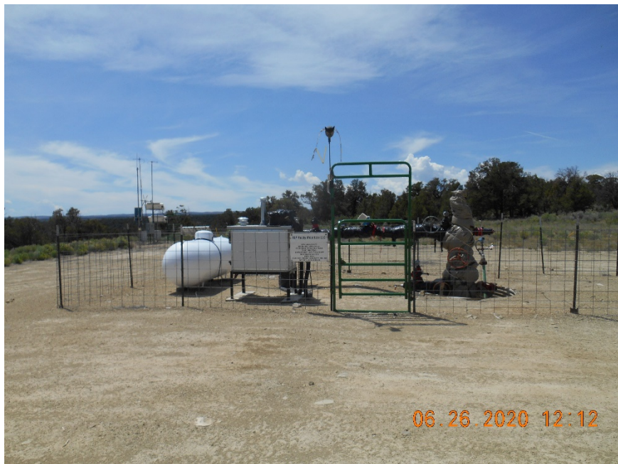
Injection wellhead & line heater
