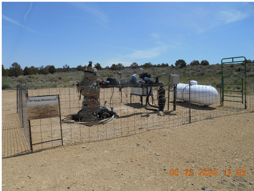
Injection wellhead & line heater
