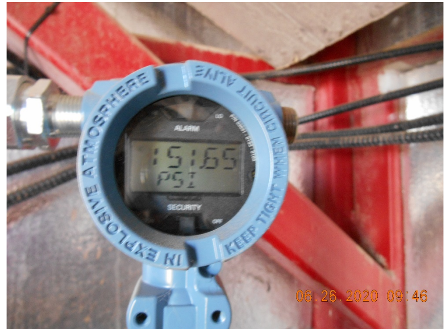
Injection Wellhead tubing gauge
