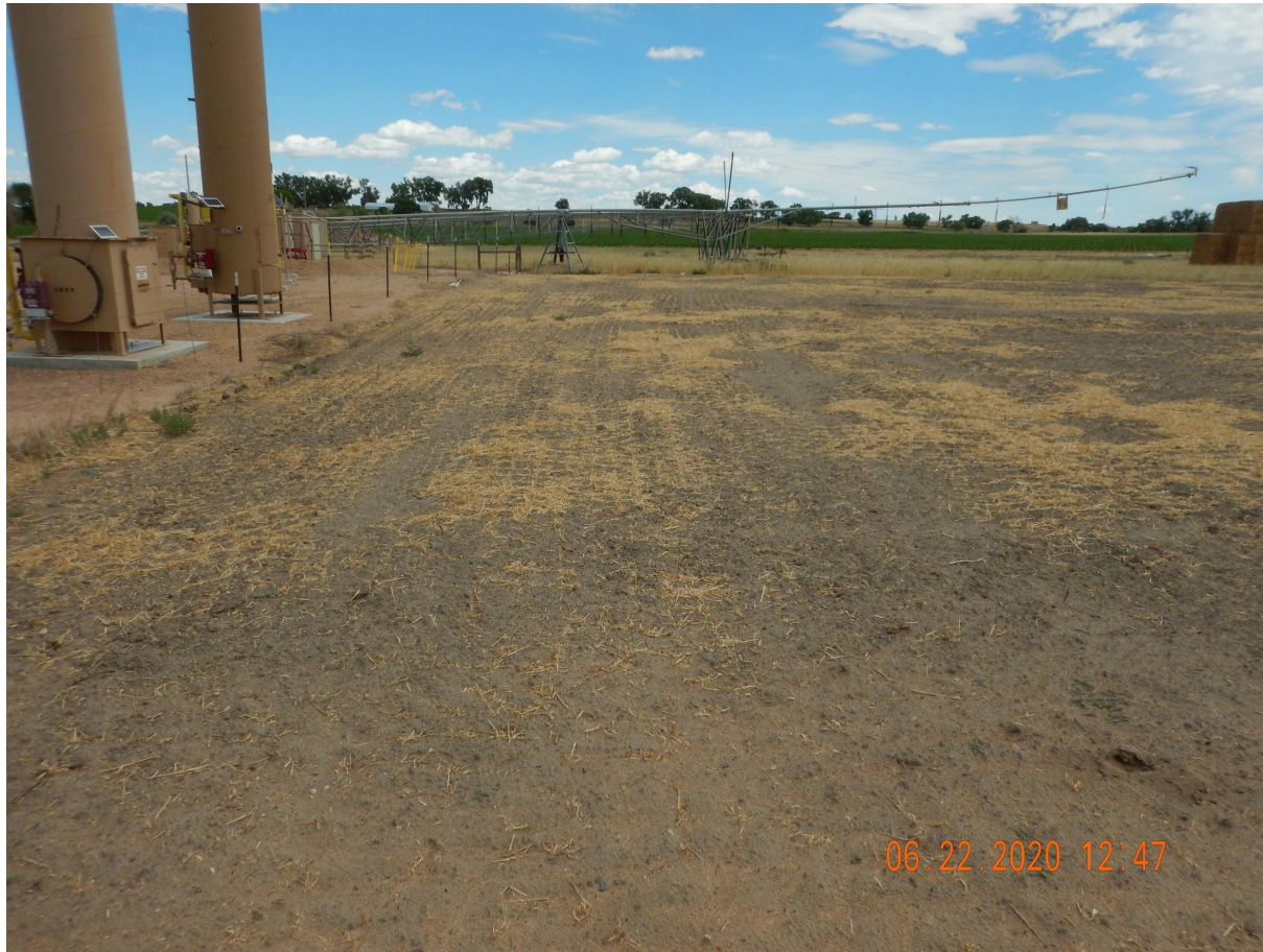
Photo 2. Photo taken from the northern portion of the flowline area, facing East. Photo illustrates the Operator has performed reclamation activities with the evidence of straw crimped mulch and drill seed rows. However, there was very little germination of any species. Note: much of the straw mulch has blown off the flowline area, which is not protecting the seeded soil from wind and water erosion. A native grass mix was believed to be planted which only gets planted \frac{1}{4} "- \frac{1}{2} " depth. Wind erosion could have potentially blown seed away.
