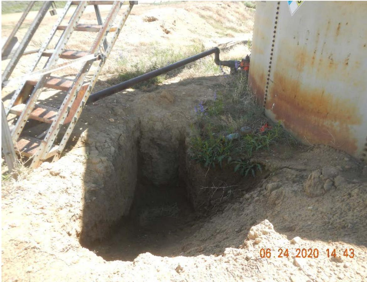
Photo #13 depression in the ground near the northern tank.
