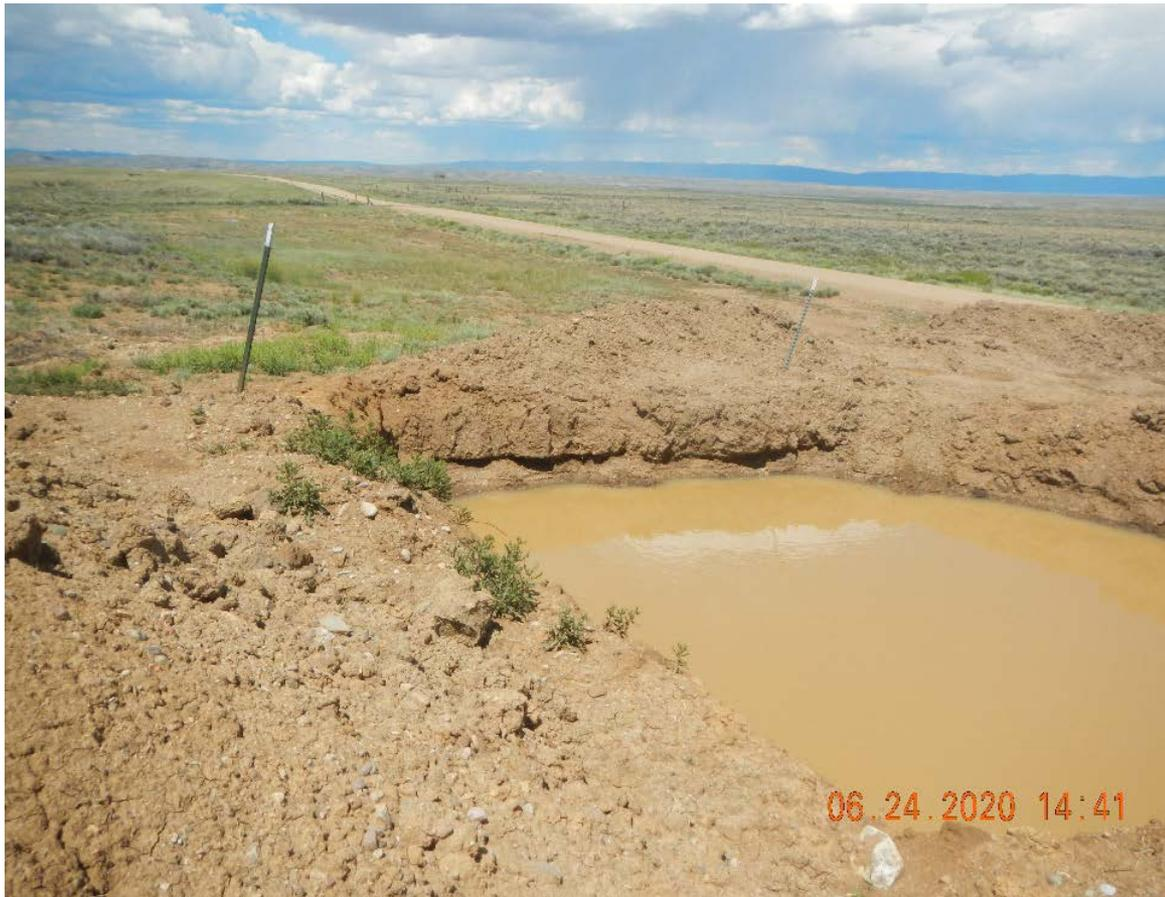
Photo #9 looking northeast. Excavation was the area of old pit and tin horn separator, is now filled with water. No obvious sign of oil (rainbows) were observed.
