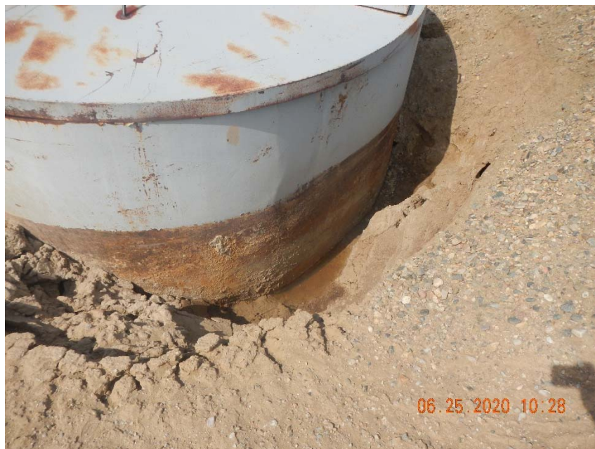
Photo 7. Hole in base of tank with water visible.
