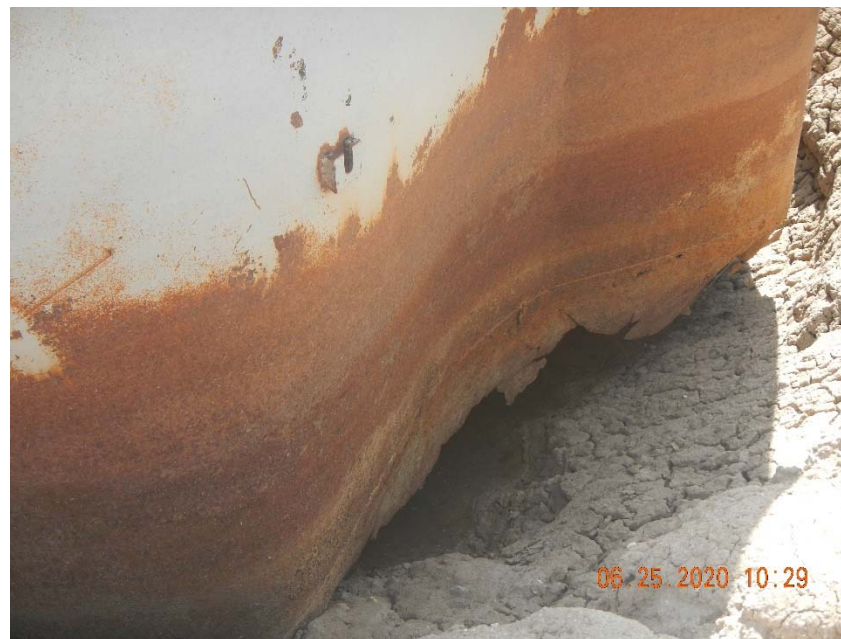
Photo 8. Close up of hole and water from photo 7.
