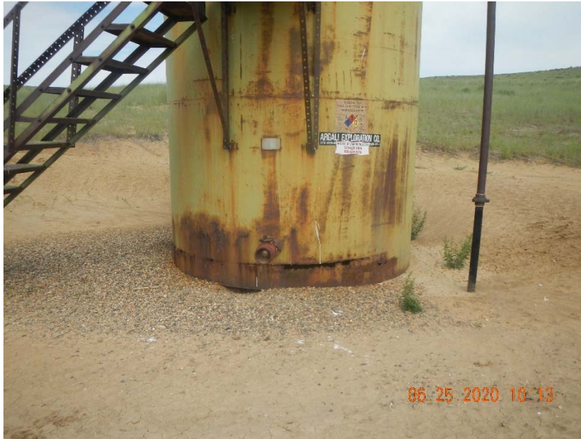
Photo 2. Holes in produced water tank.
