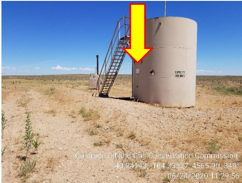
Photo 1 – Tank Battery, Weeds. Crude Oil Tank missing Content Label
