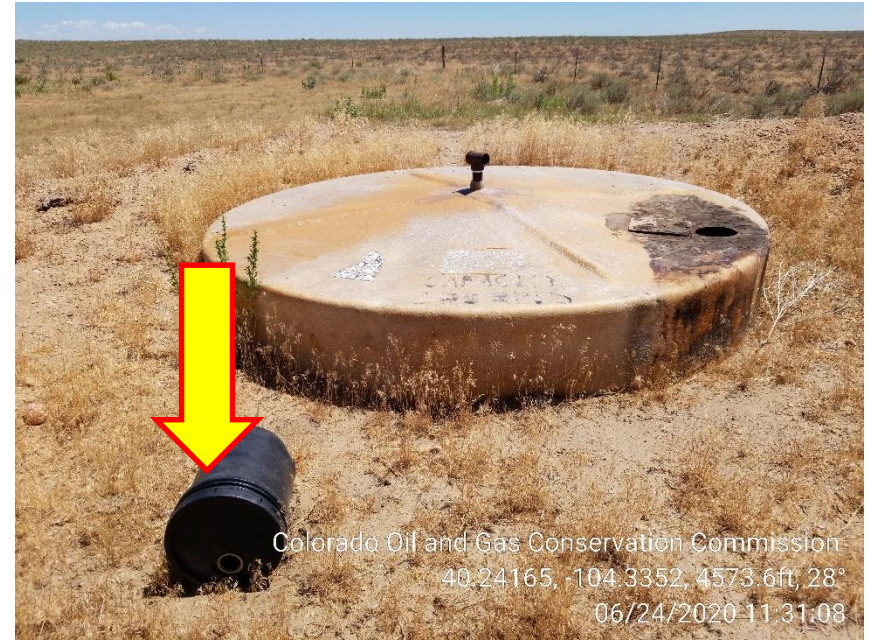
Photo 4 – Trash, Weeds. Tank missing Content and NFPA Labels
