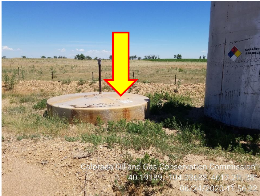
Photo 3 – Produced Water missing Content, Capacity, NFPA Labels, Weeds
