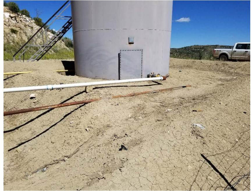
Photo #8 – Unused pipe and eroded berms on east side of tank battery.
