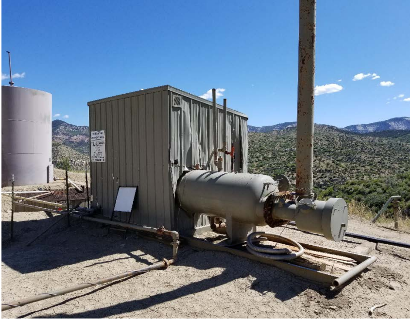
Photo #13 – View of heated horizontal separator located south of tank battery.
