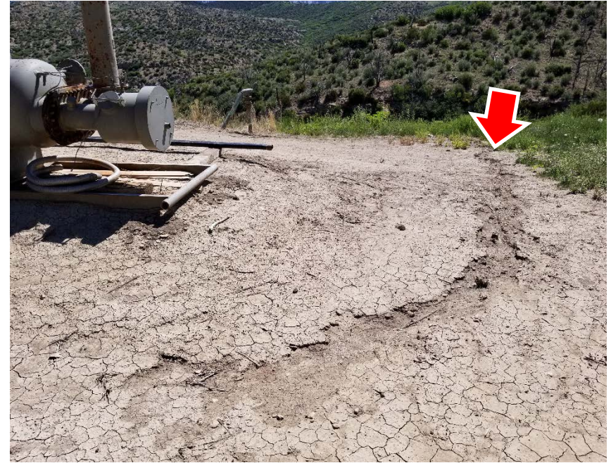
Photo #12 – Erosion feature observed in southeast corner of pad (red arrow) indicates direction of stormwater runoff.
