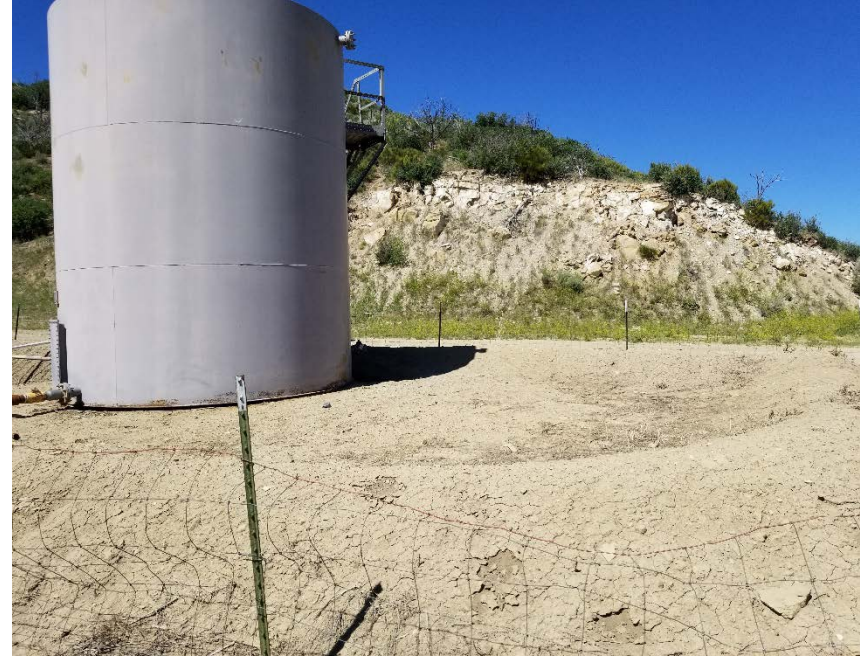
Photo #16 – View of shallow, eroded berms on north side of tank battery.
