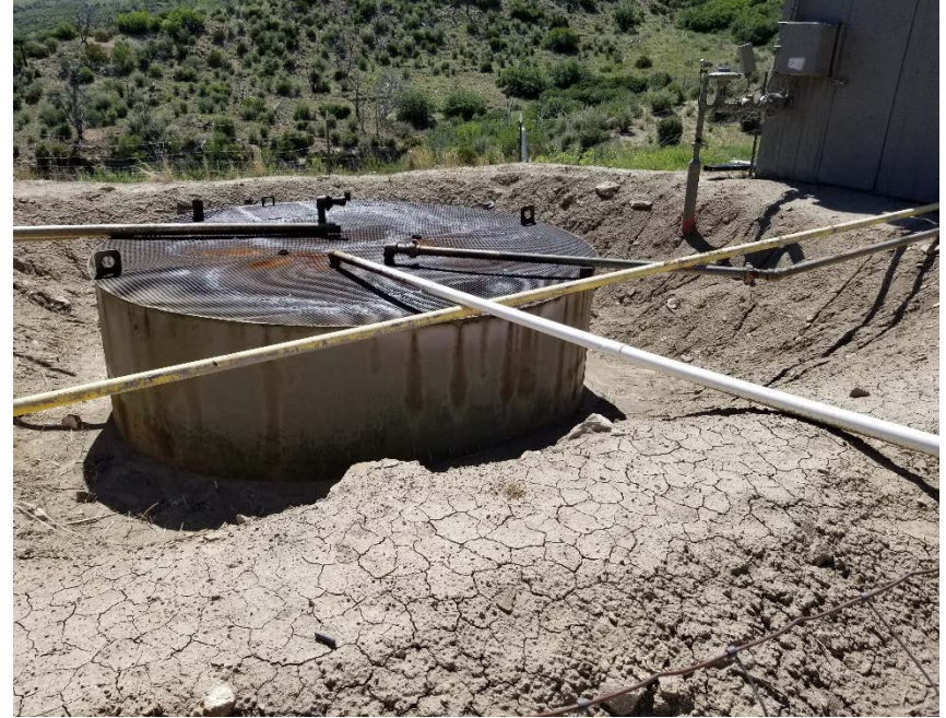
Photo #6 – View of 100 bbl fiberglass PBV skim tank from northwest. Tank is located inside of former Pit Facility ID #113000. Pit Facility status remains AC (active) in COGCC database.
