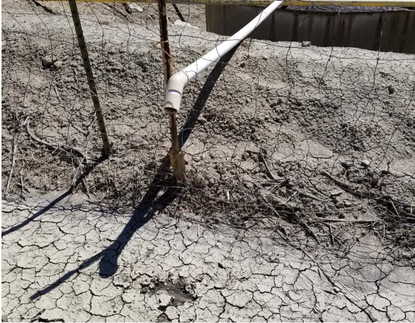
Photo #9 – Truck loadout from fiberglass PBV on west side of tank battery. Note that loadout lacks secondary containment device. Also note presence of mud cracks in loadout area is indicative of stormwater pooling in this location.
