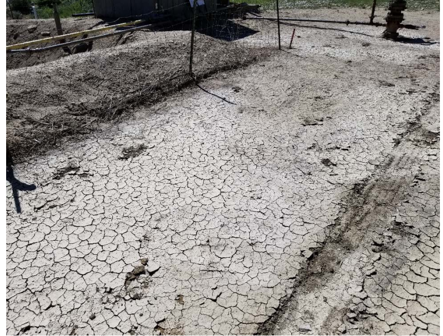
Photo #10 - Presence of mud cracks in loadout area and along west side of tank battery is indicative of stormwater pooling in this location.
