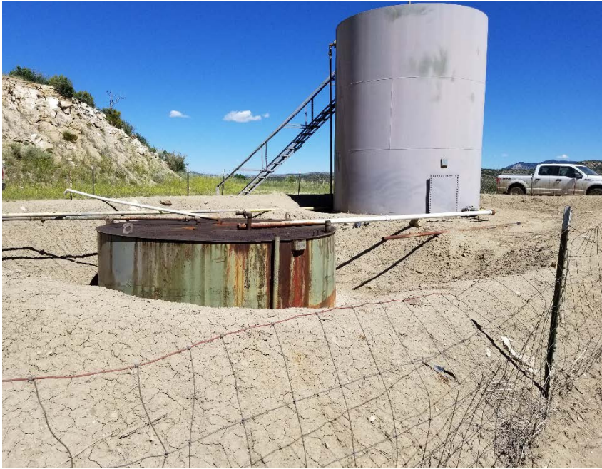
Photo #7 – View of tank battery from southeast. Note earthen berms are shallow and eroded.
