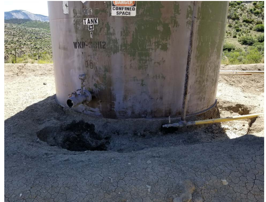
Photo #4 – Partially excavated area at base of condensate tank. Additional site investigation and remediation required in this location to address impacts from Spill #476598.
