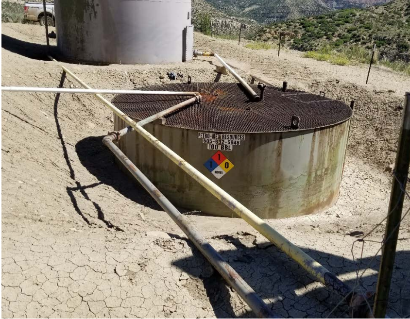
Photo #5 – View of 100 bbl fiberglass PBV skim tank from southwest. Note tank lacks content label.
