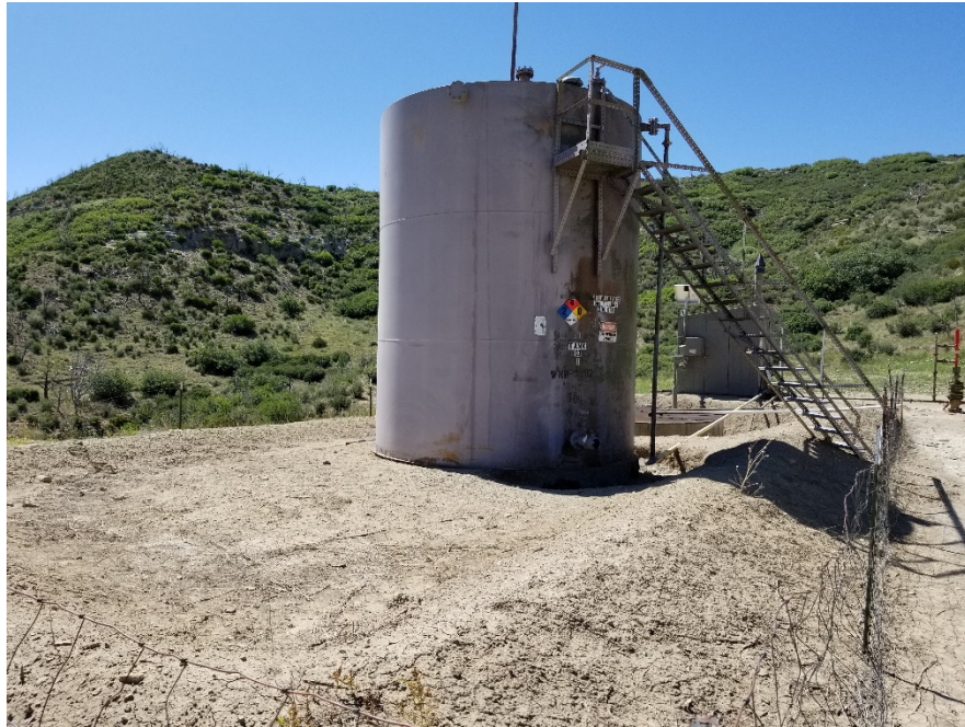
Photo #3 – View of 300 bbl condensate AST from northwest. Note berm is shallow and eroded.
