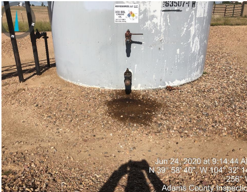
Photo #5 Stained soil under load off line of Crude tank.
