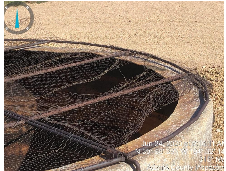
Photo #6 gaps in chicken wire over produced water tank.
