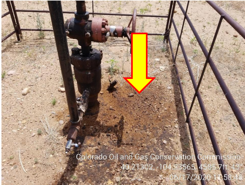
Photo 3 – Wellhead, Stained Sol
