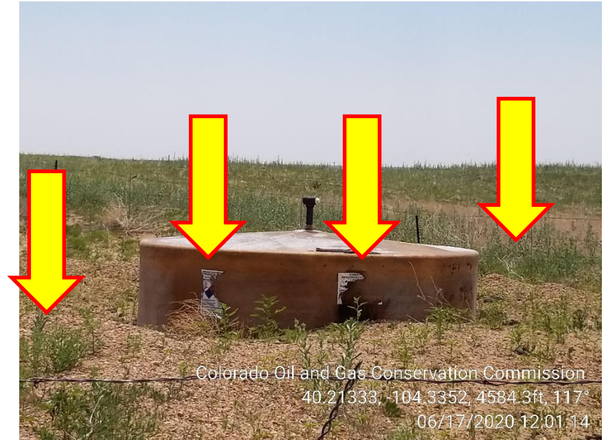
Photo 4 – Produced Water Tank – Capacity, Content, NFPA Labels missing. Weeds
