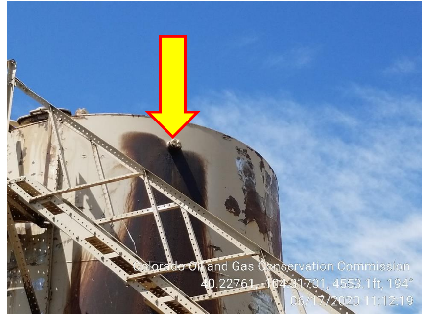
Photo 4 – Plug/Fitting leaking down the side of tank to ground
