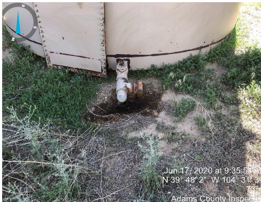
Photo #7 Stained soil next to crude tank
