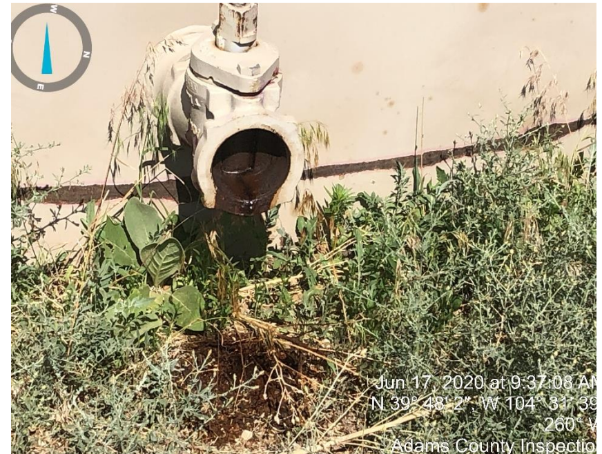
Photo #10 stained soil and no bull plug in crude tank
