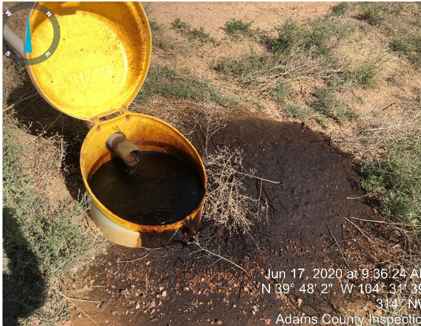
Photo #9 load off bucket full and no bull plug.
