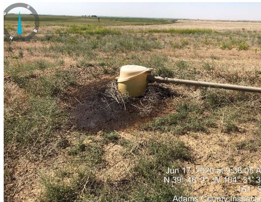
Photo #8 Stained soil around load off bucket.
