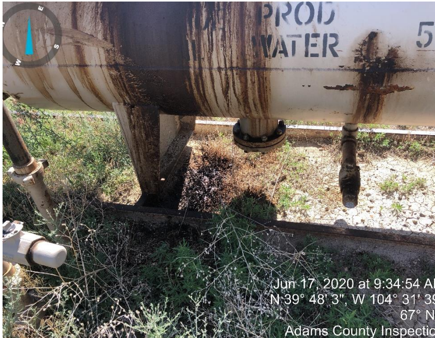
Photo #5 Stained soil under separator.
