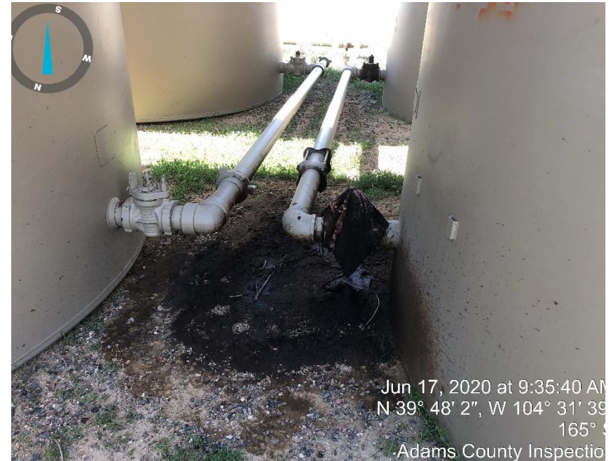
Photo #6 stained soil between crude tanks.
