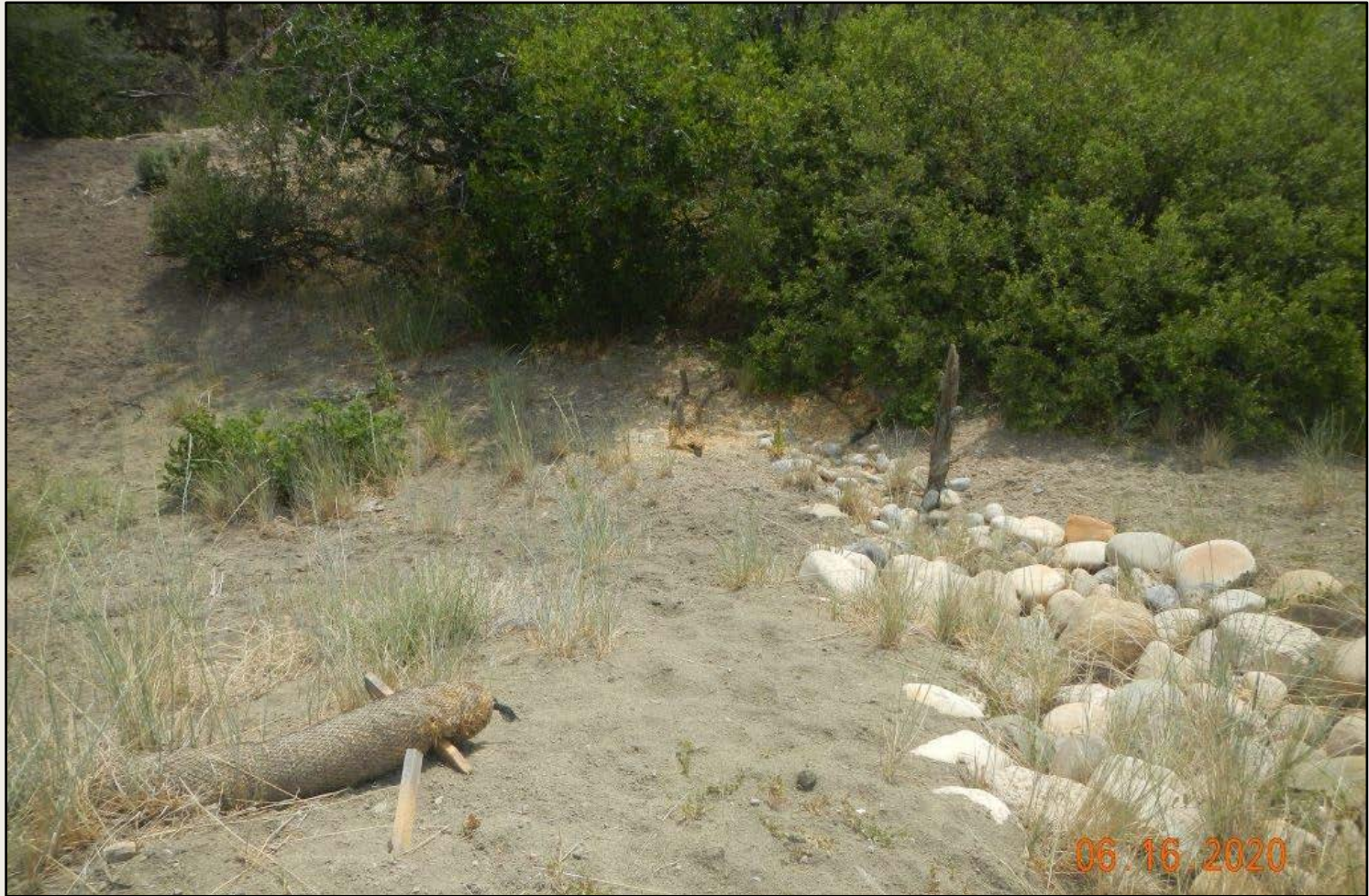
Photo 3. View of BMPs within the eastern project area that need maintenance. Wattles are no longer staked and filled with sediment, cobble run-down is filling with sediment.
