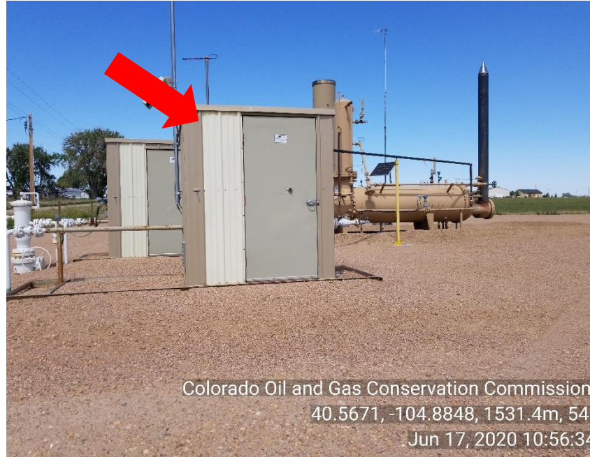
Photo 3: Disconnected/unused gas meter
