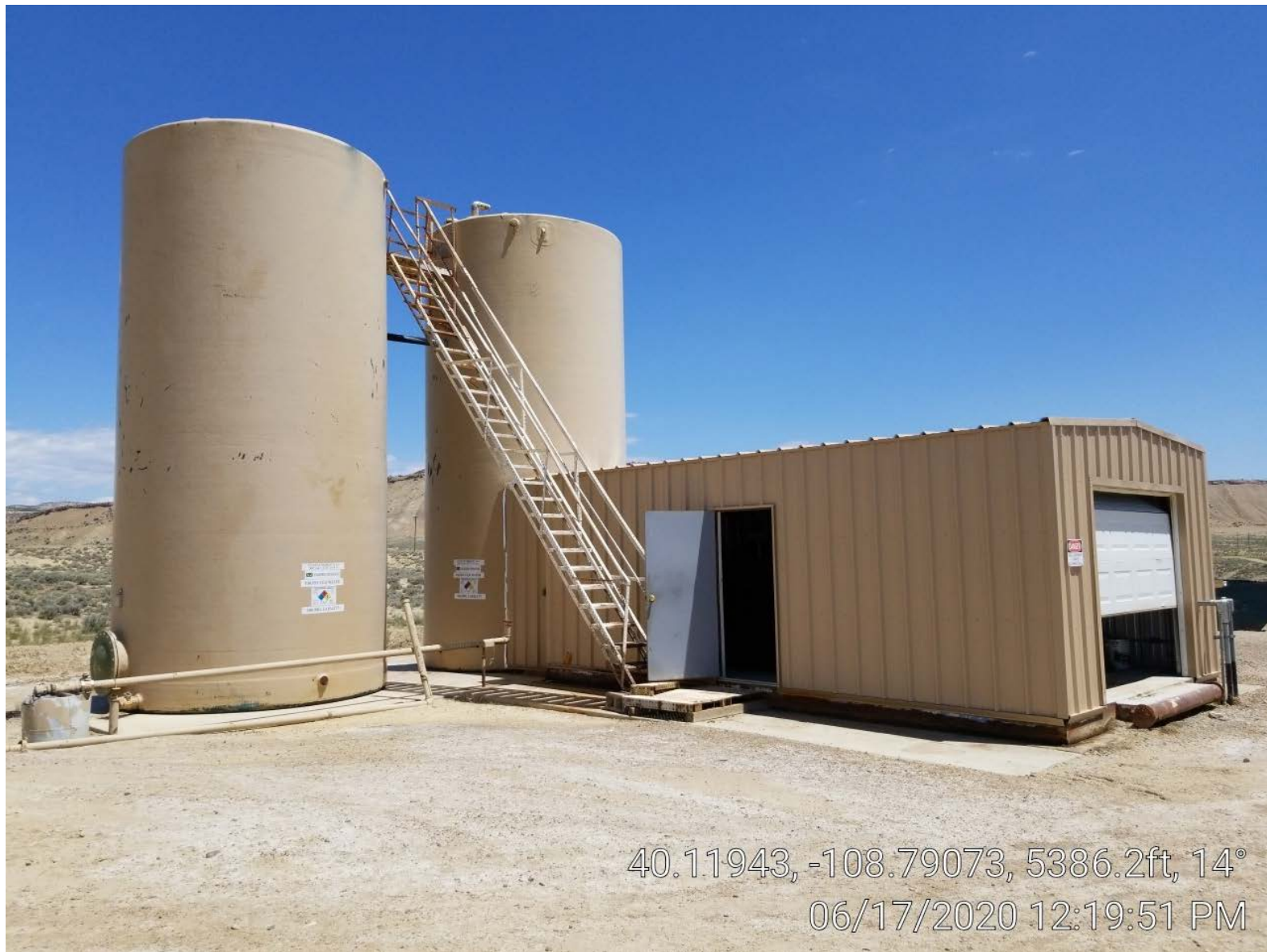
Photo 3. Produced water tanks & pump building.
