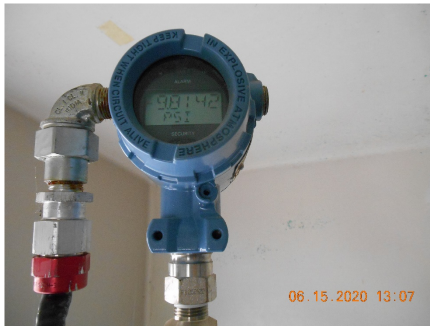
Injection well tubing gauge.
