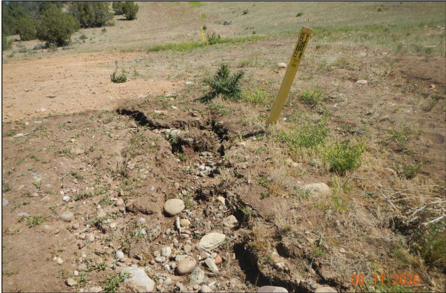
Photo 5. View of erosional channel approximately 1.5 feet wide and 8 inches deep, near the well pad entrance.
