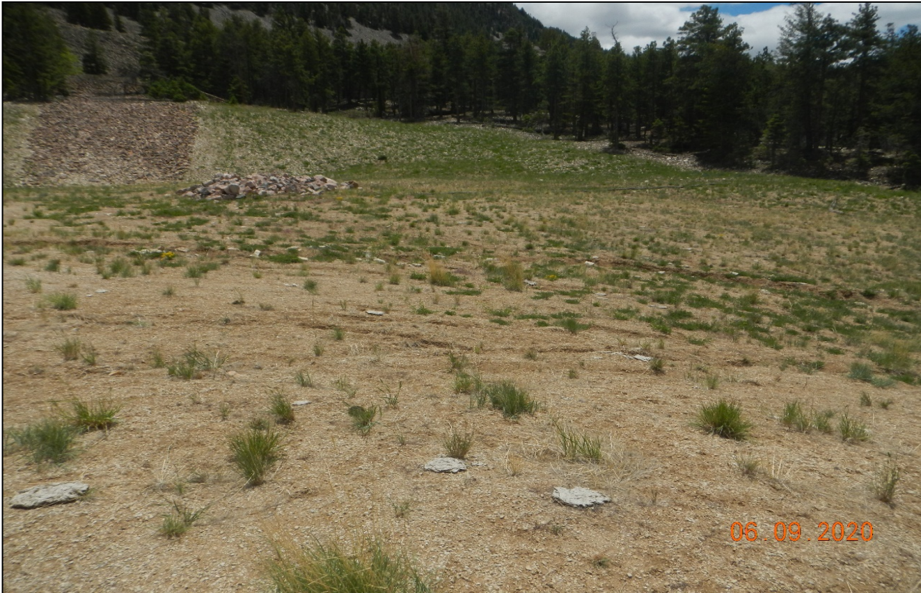
Photo 3. Facing southeast toward the interim reclamation area. Vegetation has not adequately reestablished and there are signs of erosion.
