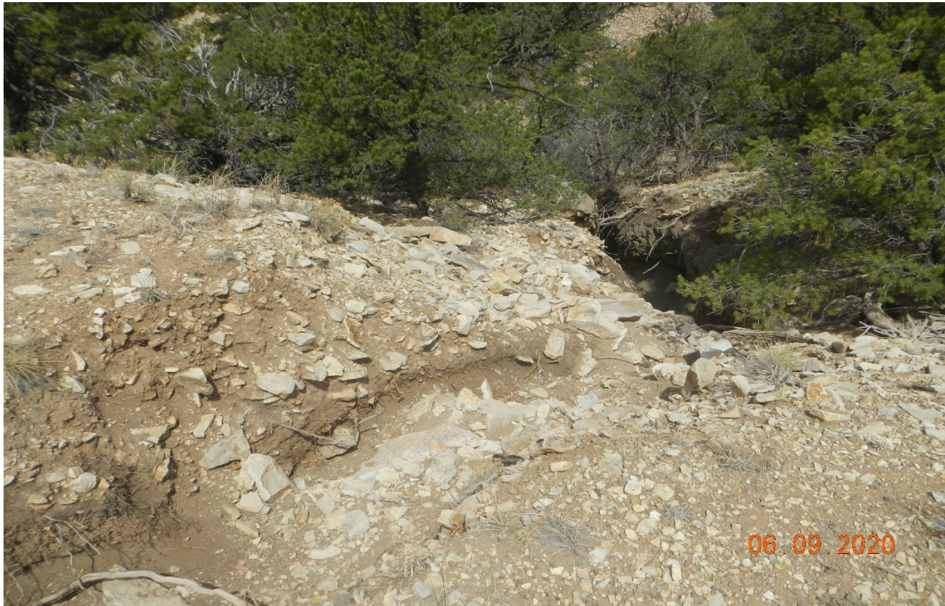
Photo 4. Facing nothwest toward erosion which is occurring from stormwater runoff shown in previous photo at Lat/Long:37.71484,-105.23178.
