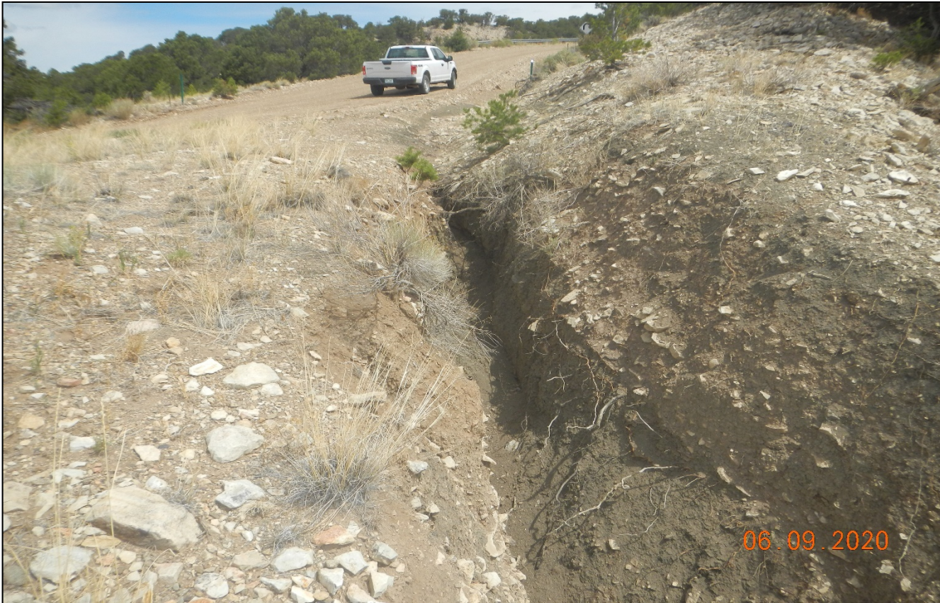
Photo 1. Facing north toward the access road. There is erosion occurring caused by stormwater directed off the road at Lat/Long:37.71484,-105.23178.
