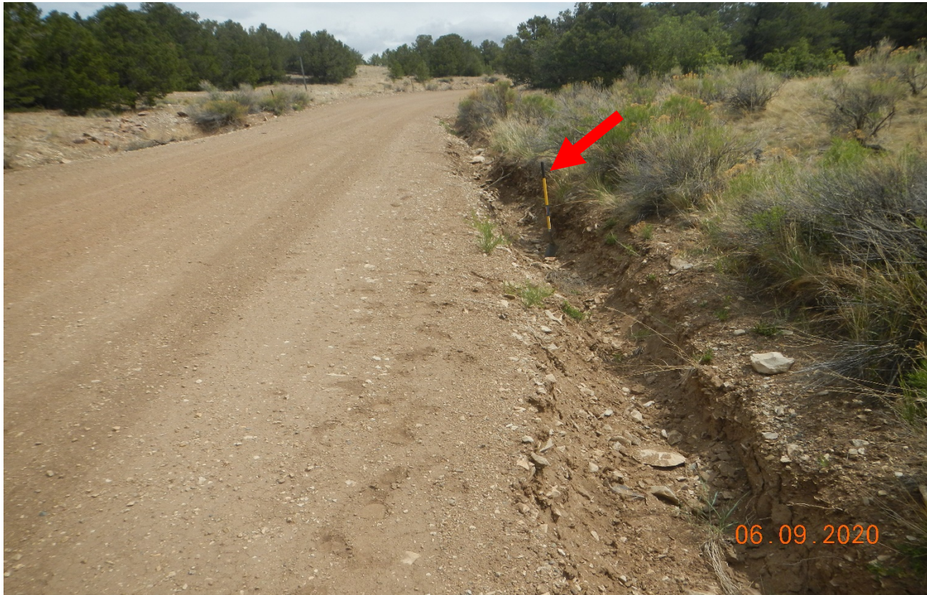
Photo 5. There is erosion occurring along the main access road at Lat/Long:37.71665,-105.22713. Red arrow points to 4.5 ft. shovel to depth of erosion.
