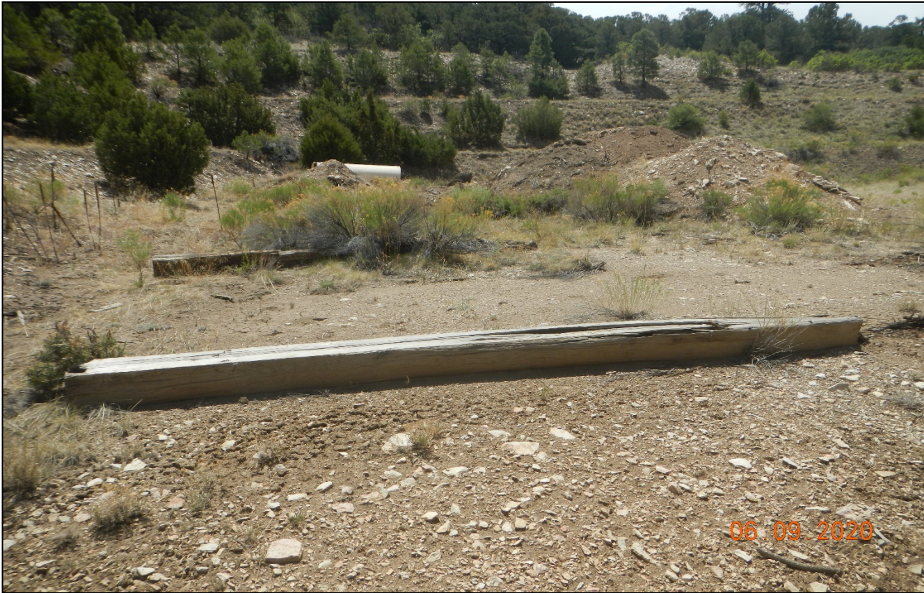
Photo 10. There is degraded wood timbers that need to be removed.
