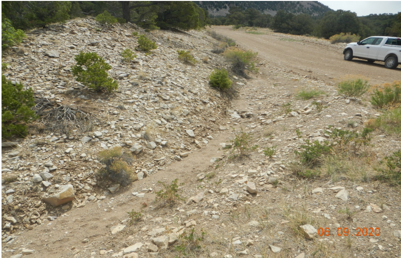
Photo 3. Facing east on the next switchback of the road. Stormwater is directed off the road which is causing erosion shown in the next photo at Lat/Long:37.71576,-105.23161.
