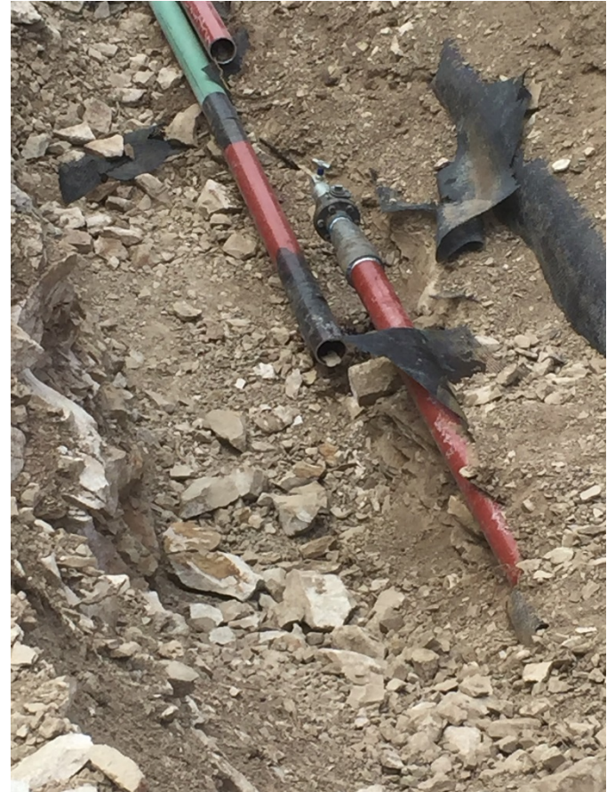
Flowline cut and future pressure test from here to can, plan forward will be made with results of pressure test
