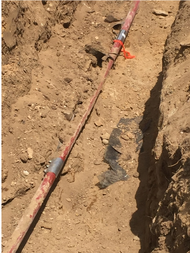
Produced water gathering flowline with 2 temporary patches installed for pressure test
