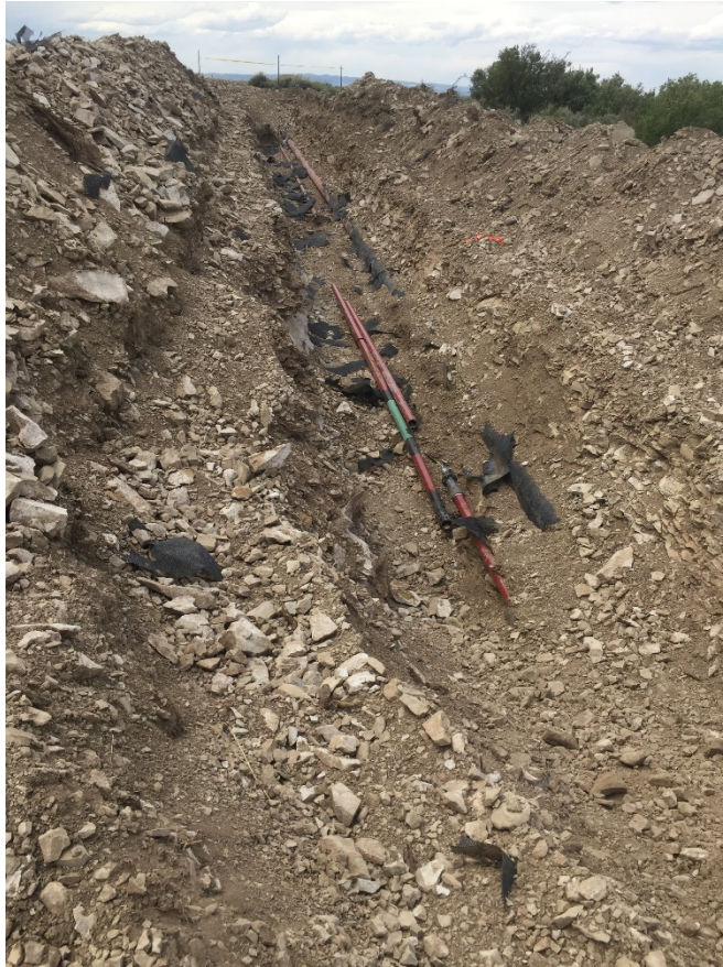
Produced water gathering flowline with 2 temporary patches installed for pressure test at 2 nd excavation site
