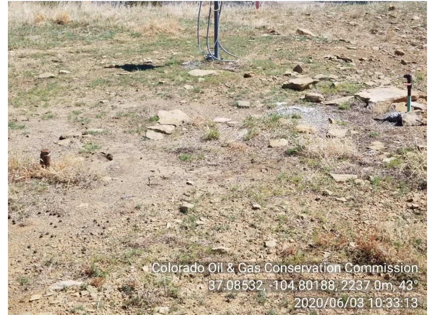
PHOTO 4: UNUSED EQUIPMENT (ONE 2" RISER AND ONE 1" RISER). REMOVE UNUSED EQUIPMENT COMPLY WITH NTO AND RULE 603.f. ca date 9-3-20
