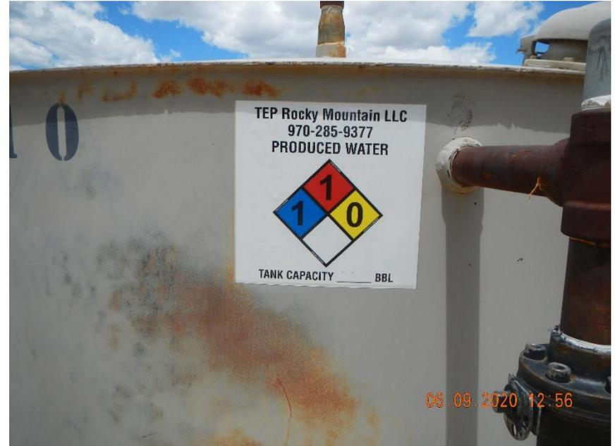
**Tank capacity is blank on label.**
