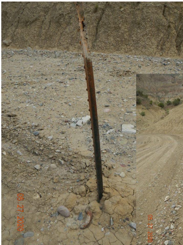
Photo#6: Anchors need maintenance.
