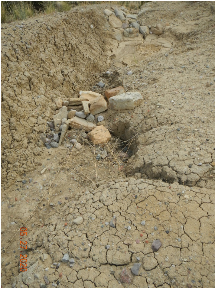
Photo#4: Erosion, undercutting of BMPs.
