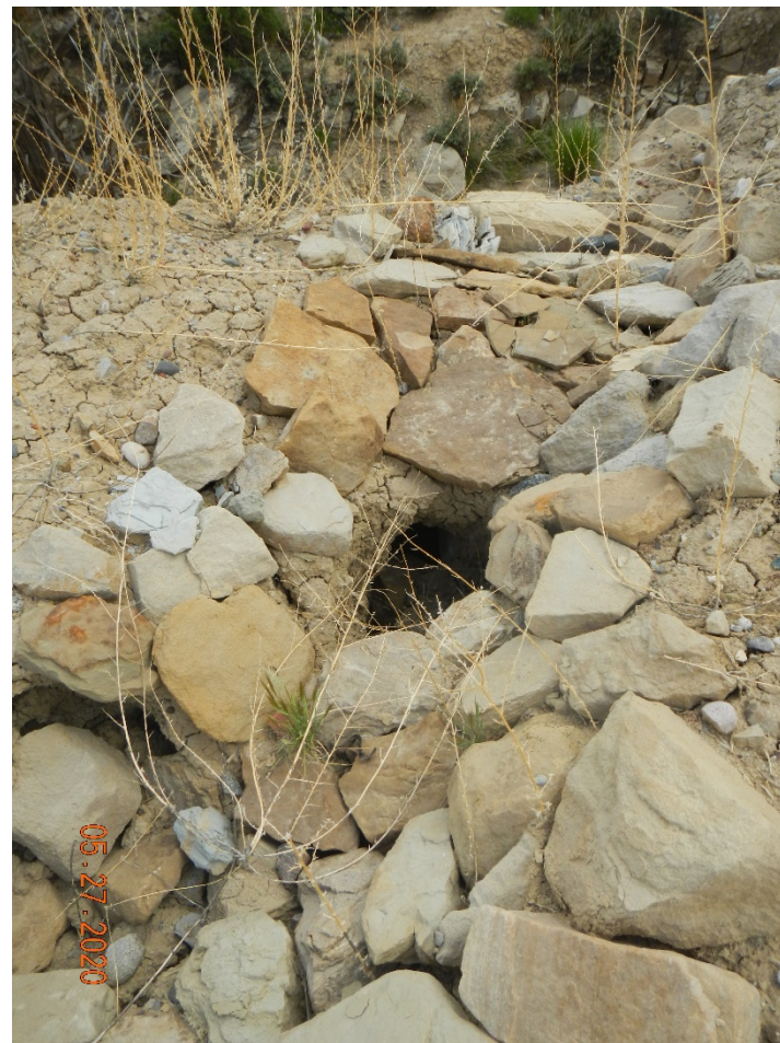
Photo#3: Erosion, undercutting of BMPs
