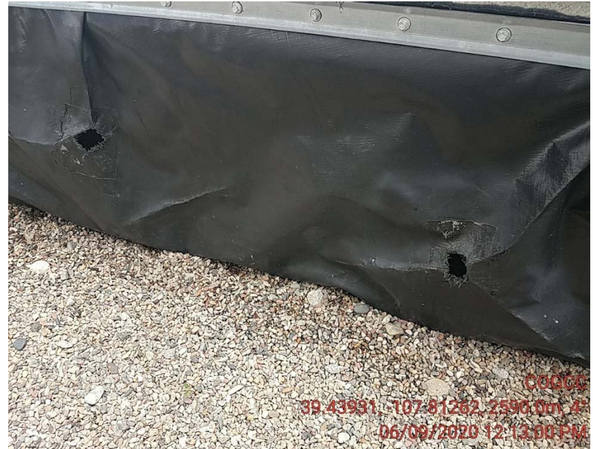
Holes in containment
