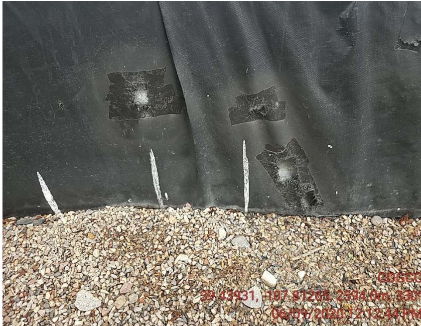
Holes in containment
