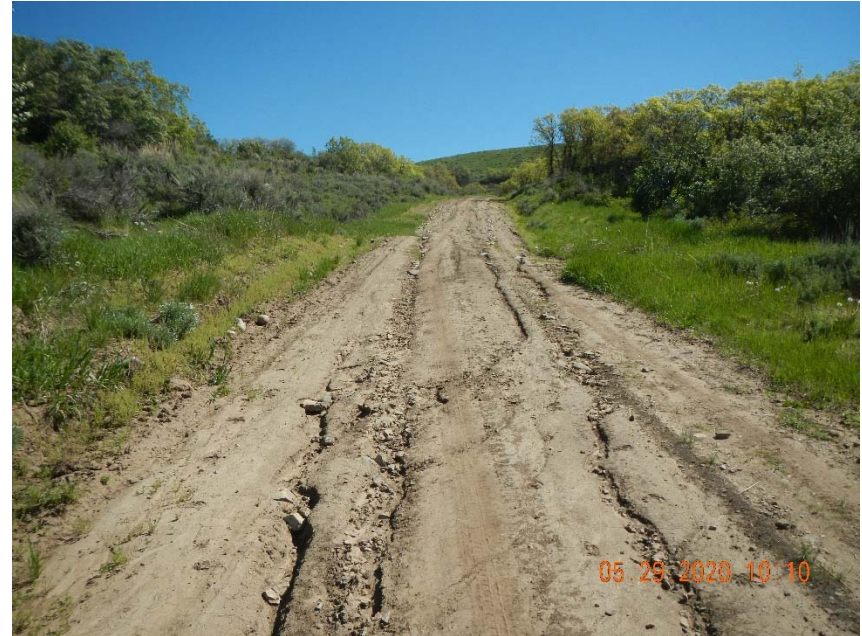
Photo 5. Example of rills on access road.
