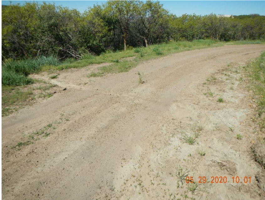
Photo 6. Example of sediment being transported onto and across access road.
