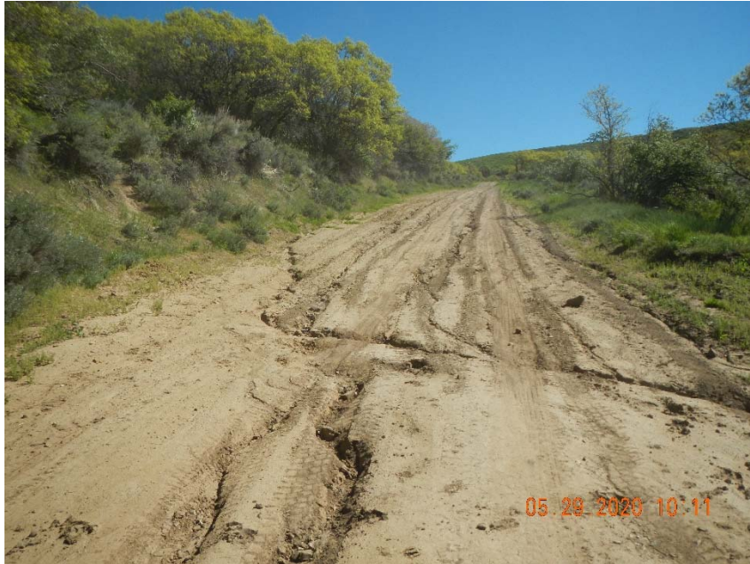
Photo 4. Example of rills on access road.
