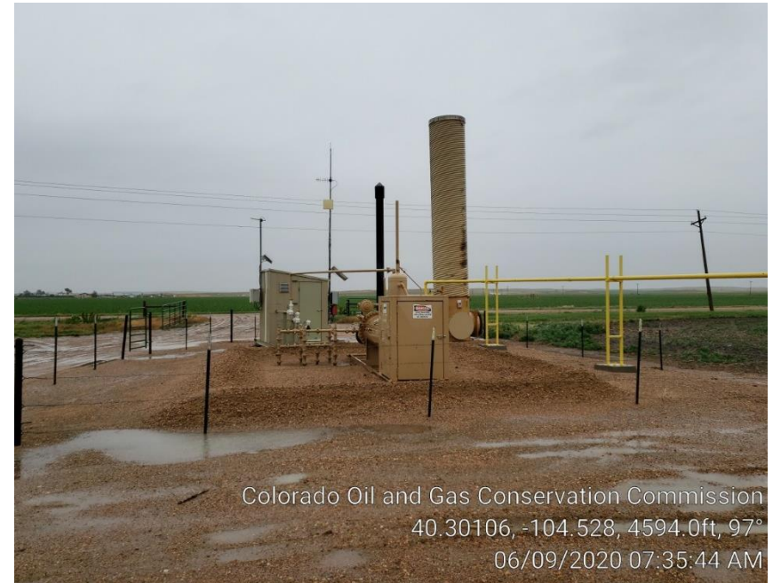
Photo #2 Separator, ECD & Meter Run
