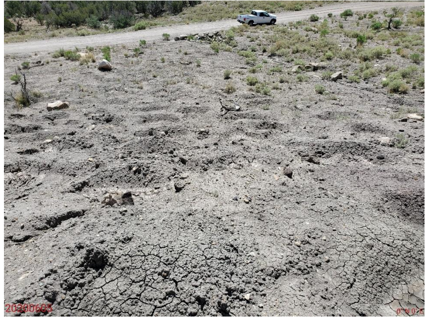
Photo 2: Photo taken from the west end of the Location, facing east. Photo provides overview of the Location. Photo also shows previously observed erosion concerns have been repaired and pitting has been installed; Unclear if revegetation activates have been conducted; BMPs appear insufficient to stabilize slopes.
