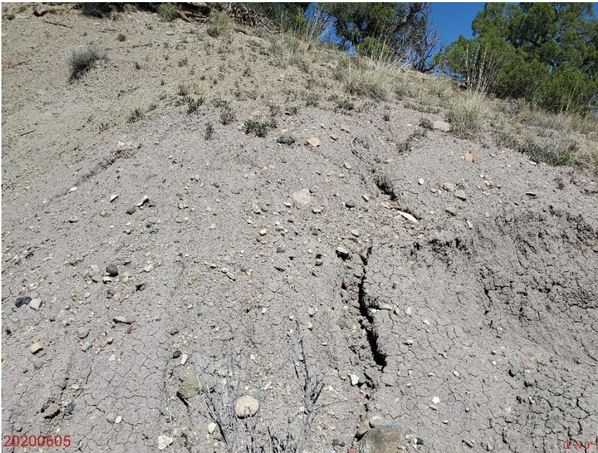
Photo 3: Photo taken from the Slopes of the Location; Photo shows erosion degradation (rilling) is recurring.
