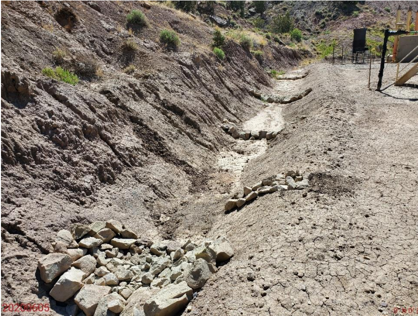
Photo 3: Photo shows additional armoring has been placed within ditch.
