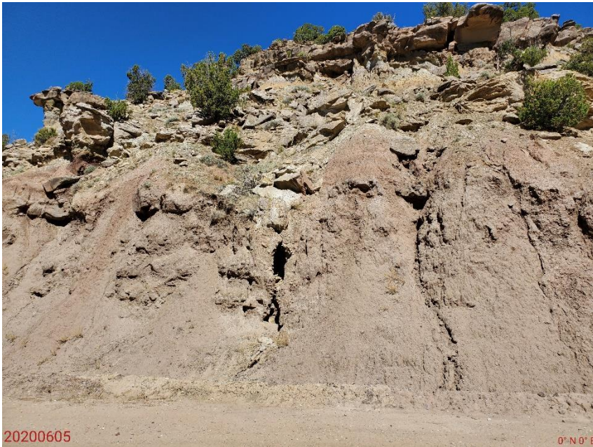
Photo 1: Photo taken from the west end of the Location, facing west. Photo shows BMPs remain insufficient or missing; stormwater runoff has caused erosion degradation on the slopes, cutting into the hillside; Water appears to be undercutting large rocks; potential rockfall risk.
