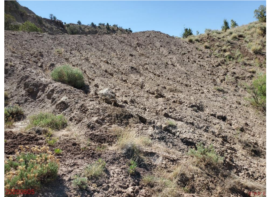
Photo 4: Photo taken from the east end of the Location, facing east. Photo shows erosion degradation on slopes; BMPs to stabilize and protect slopes remain insufficient or missing.
