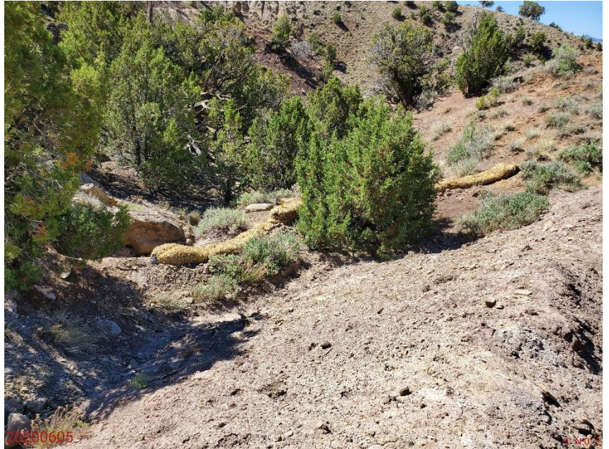
Photo 6: Photo taken from the slopes on the east end of the Location, facing east. Photo shows Operator has installed straw bales to prevent sediment deposition off location.
