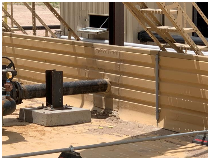
Photo 3 – Repair of secondary containment wall where pipeline breached containment wall. Patch sealed and secured with screws and then the entire repair area recoated with sealant.
