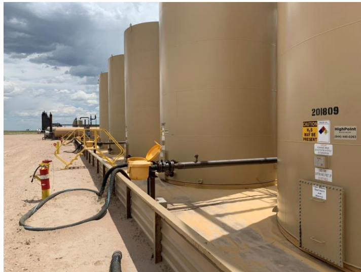
Photo 2 – View toward the east showing load point and secondary containment in vicinity of produced water tanks and load point.
