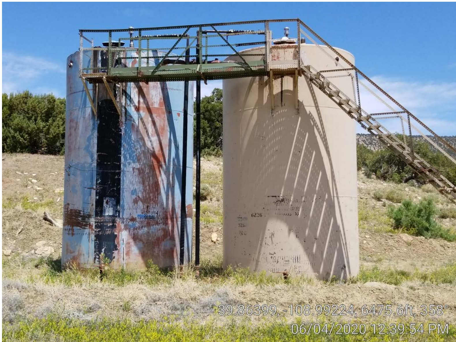
Photo 2. Tank battery.
