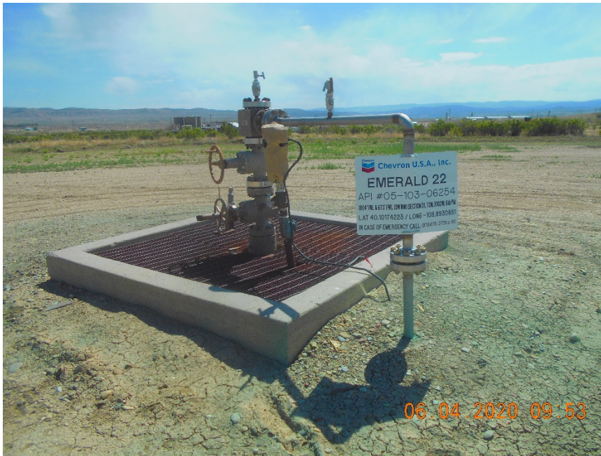
Injection wellhead.
