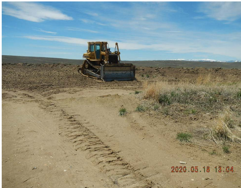
Dozer in cell 1. All cells recently ripped and turned. Slight hydrocarbon odors noted in soil in cell 1.
