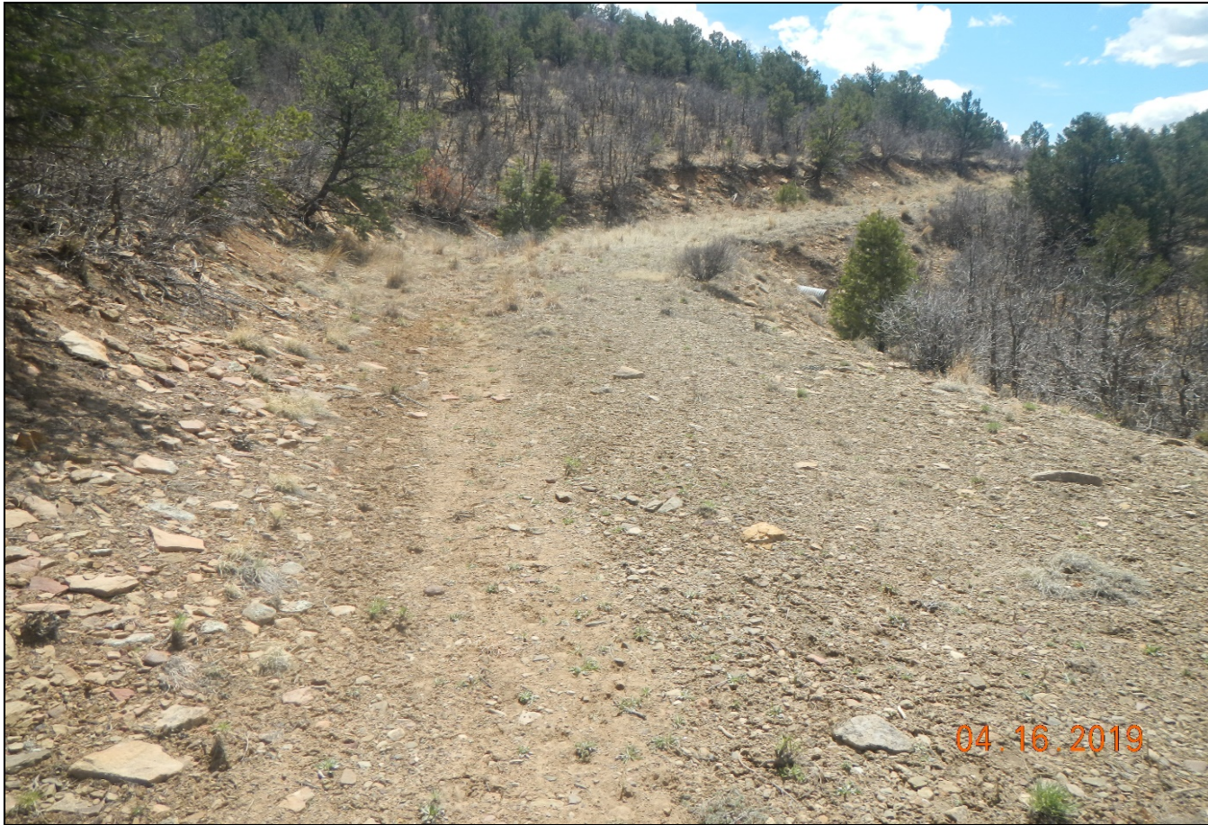
Photo 4. Further along the road. Access road has not been recontoured and reclaimed.
