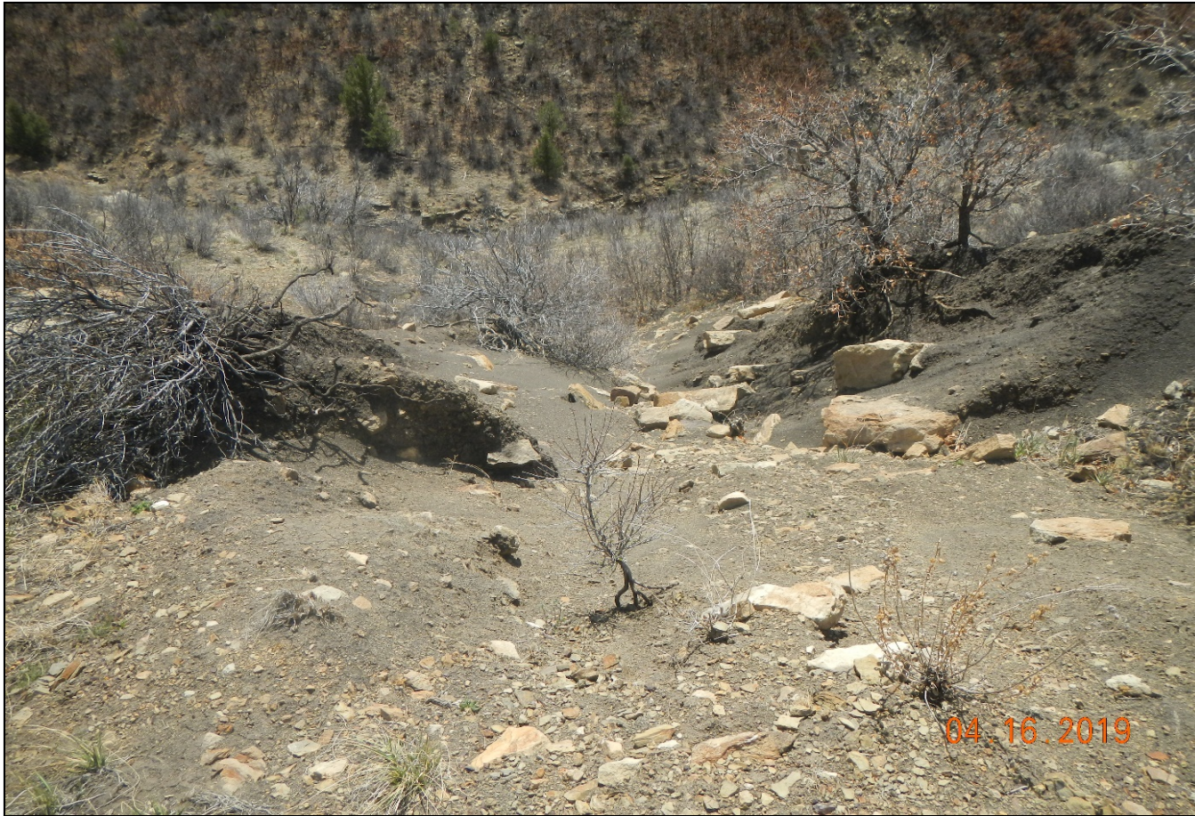
Photo 10. There is significant signs of erosion off the southeast fill slope.
