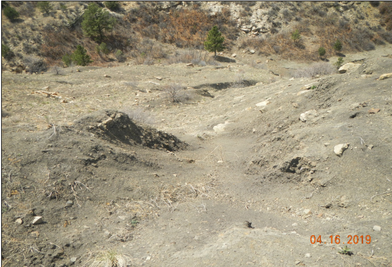
Photo 8. Facing down the fill slope shows signs of erosion.
