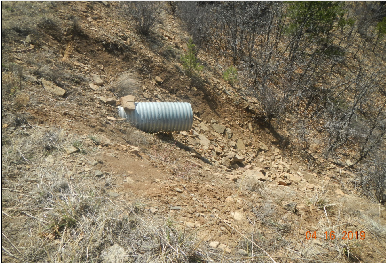
Photo 5. Culvert remains along the road. Erosion is occurring around the outlet.
