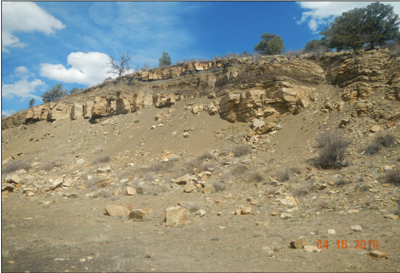
Photo 12. Facing towards the unstable vertical cut slope. Estimated to be 75' high.
