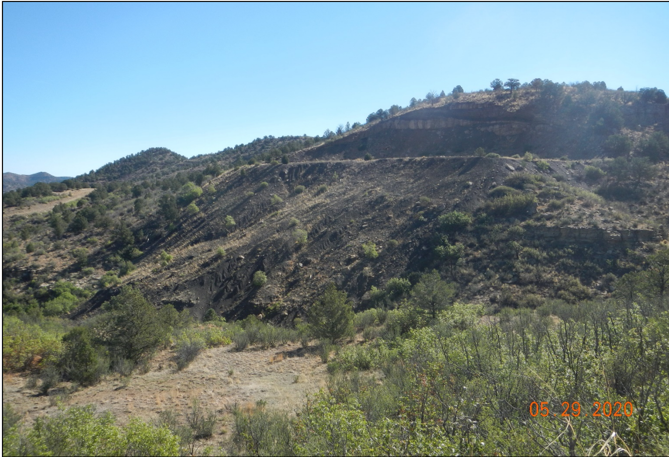
Photo 13. Facing east toward the location from across the canyon. The fill slope is not stabilized and shows signs of erosion. Location not recontoured. Photo taken 5/29/2020.
