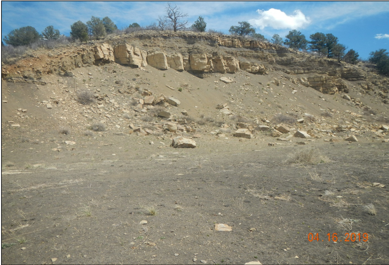
Photo 7. Facing towards the unstable vertical cut slope. Estimated to be 75' high.
