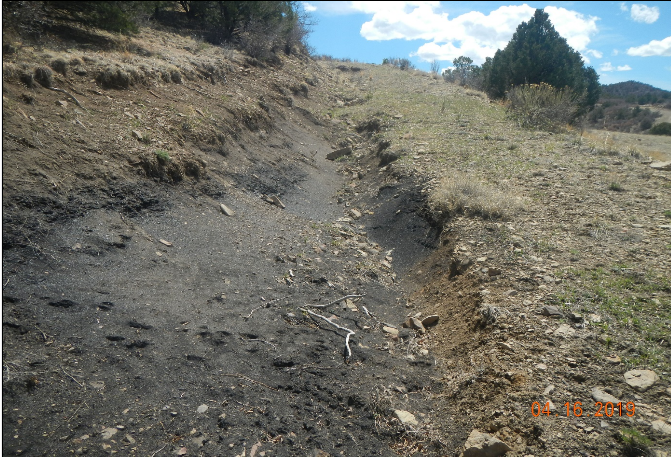
Photo 3. Photo shows erosion along the access road. Access road has not been recontoured and reclaimed.
