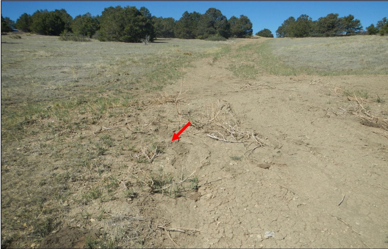
Photo 10. Facing southwest along the access road ascending toward the location. Water bars are installed along the road. This one can use minor maintenance as signs of stormwater are shown at red arrow.
