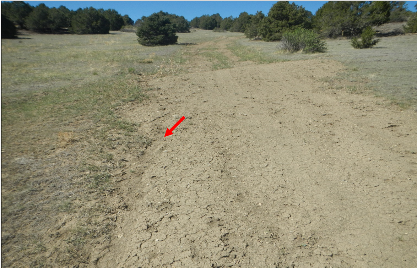
Photo 9. Facing southwest along the access road ascending toward the location. Water bars are installed along the road. This one can use minor maintenance as signs of stormwater are shown at red arrow.
