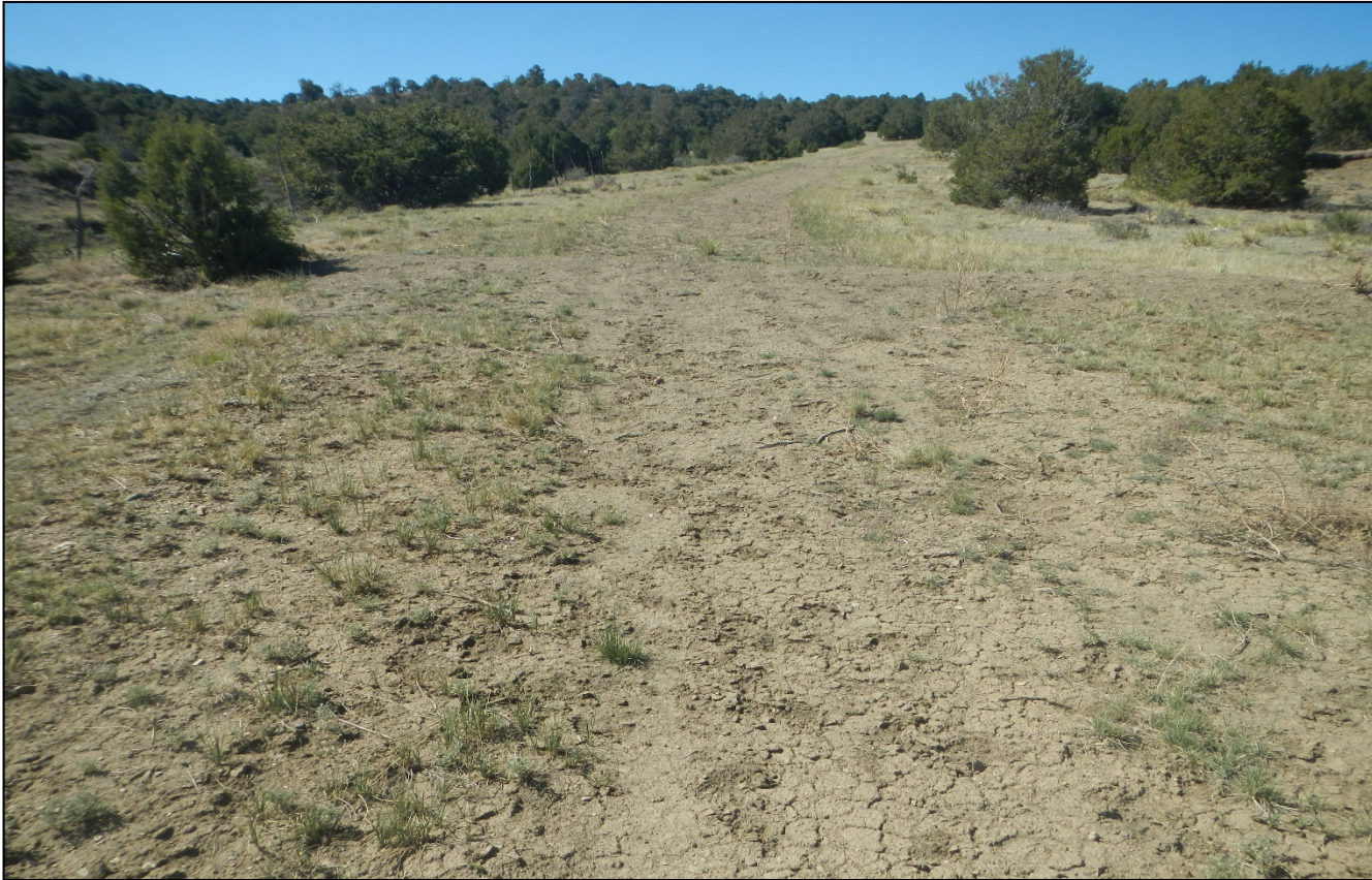
Photo 6. Facing south along the access road. This water bar/berm has been installed along the road which extends out toward the right of the photo. The area to the right is shown in the next photo.
