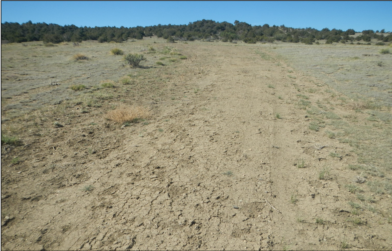
Photo 5. Facing south along the access road. Areas of erosion along the road previously observed have been repaired and appear to be stabilized.
