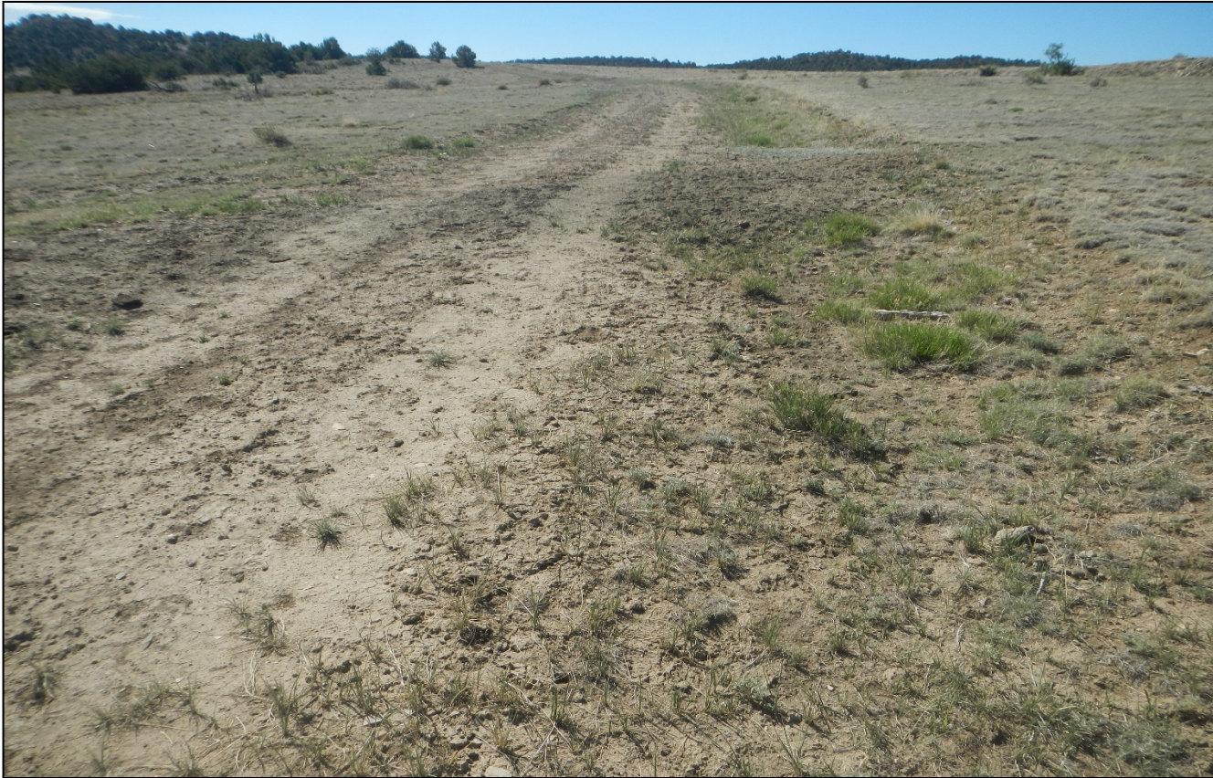
Photo 3. Facing southeast along the access road. There are water bars installed along the road to divert stormwater off the road.
