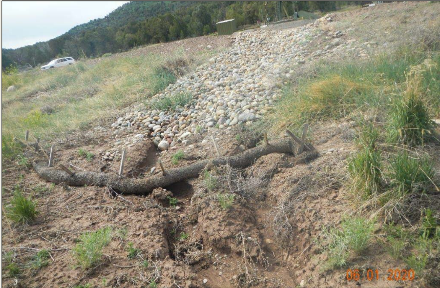
Photo 2. View of erosional channeling occurring downstream from cobble BMP in the northern project area. Wattle is failed. Cobbles are not sufficient to stabilize stormwater flows in this area.
