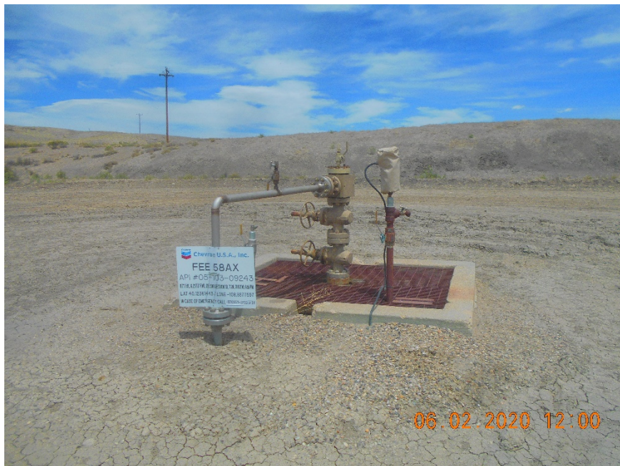
Injection wellhead.
