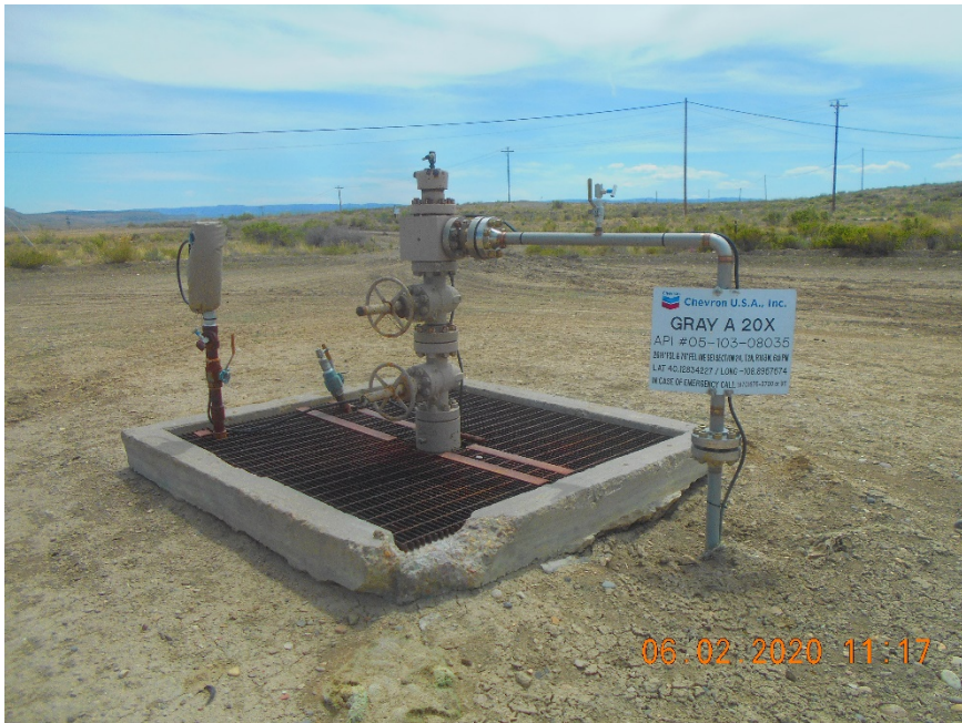
Injection wellhead.
